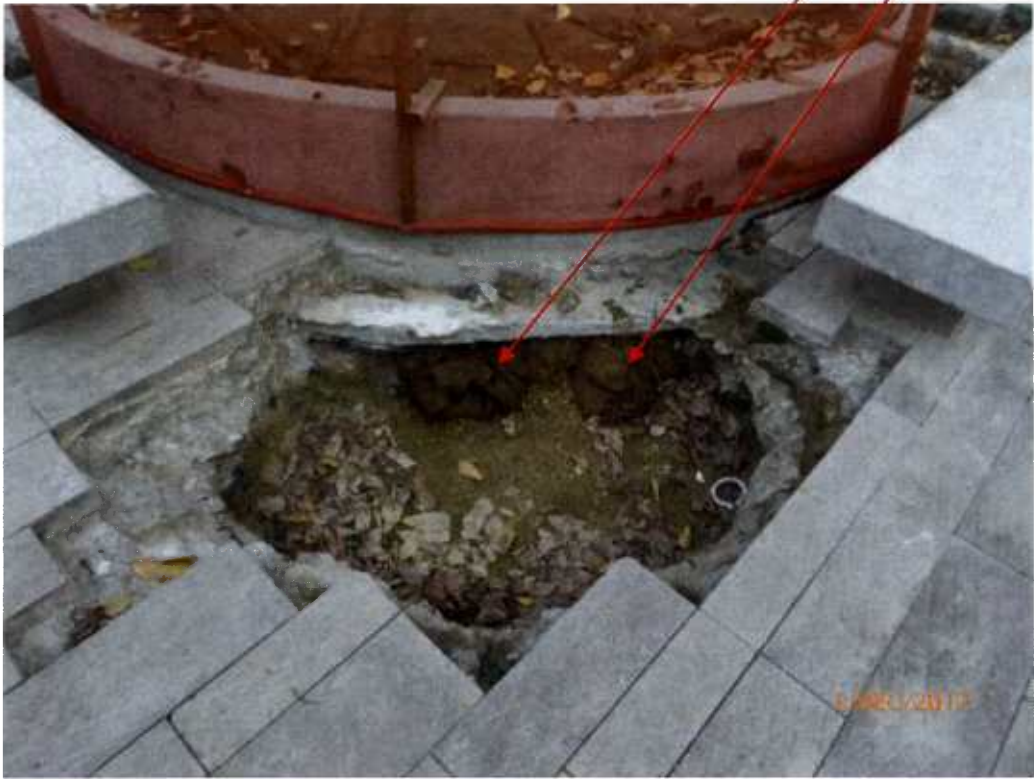
Fig. 10 The bare roots at the pits have been wrapped with hessian clothes .
