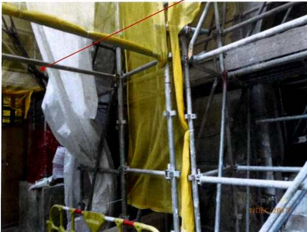
Fig. 11 Renovation works are in progress near Tree 11
