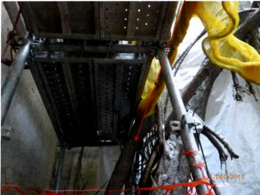
Fig. 9 A large working platform is set up close to Tree-11 .
