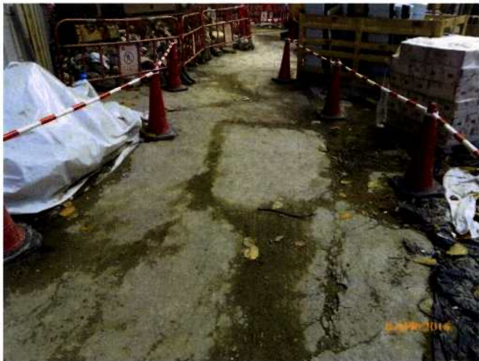
Fig. 11 The access outside the cordon zone appears clean and tidy.
