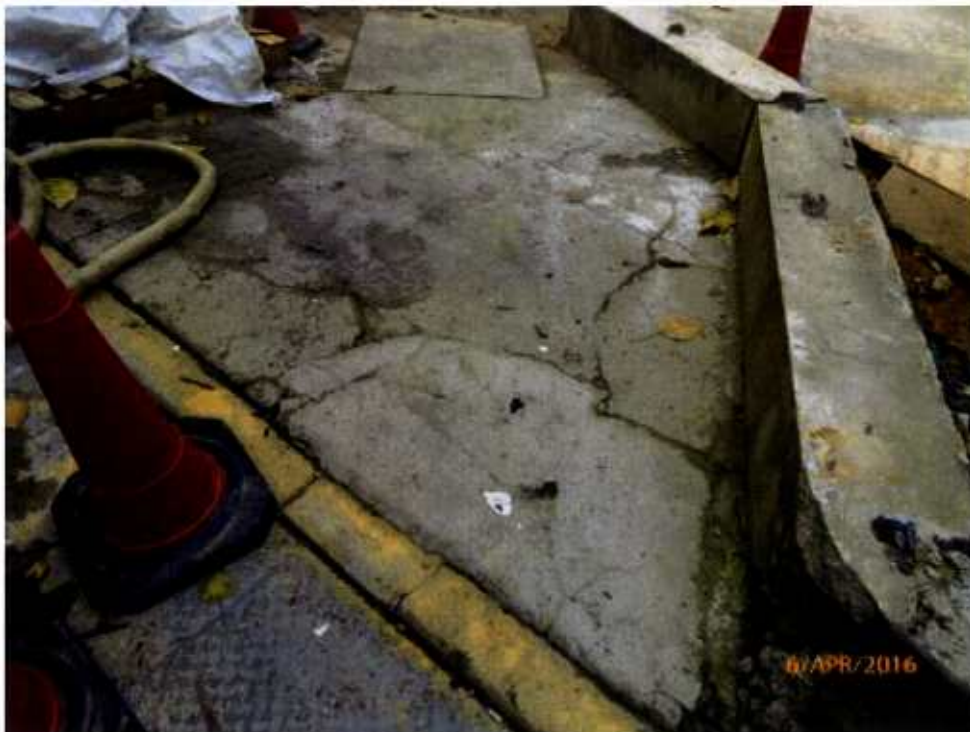
Fig. 9 The access near the tree appears clean and tidy.
