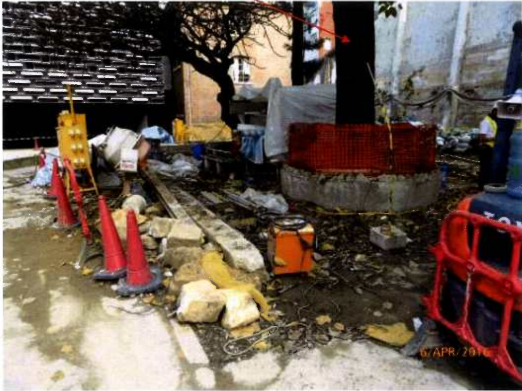
Fig. 10 The site near Tree-7 is under renovation.
