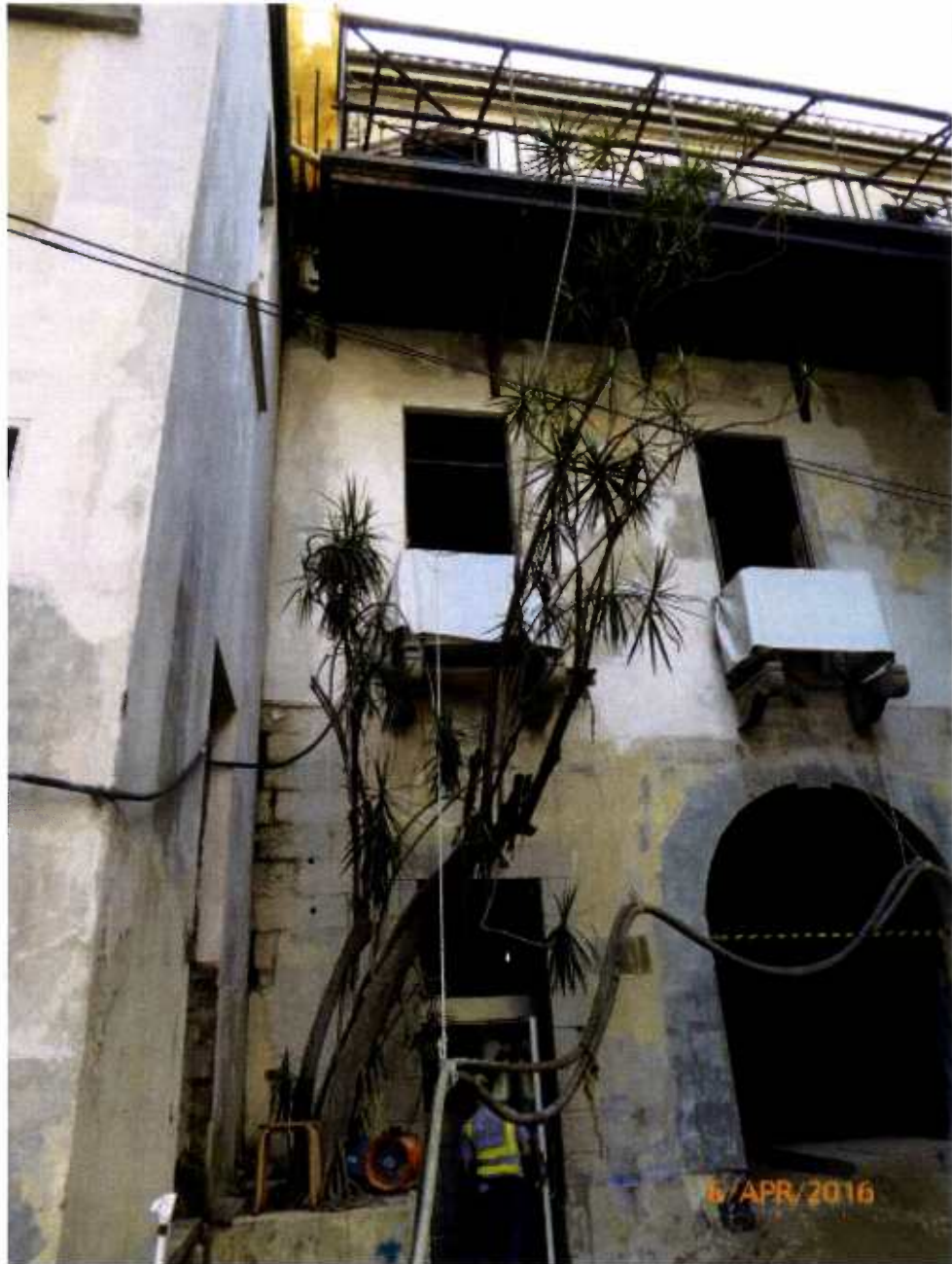
Fig. 12 Overall view of Tree 11 during inspection on 6 th April 2016.
