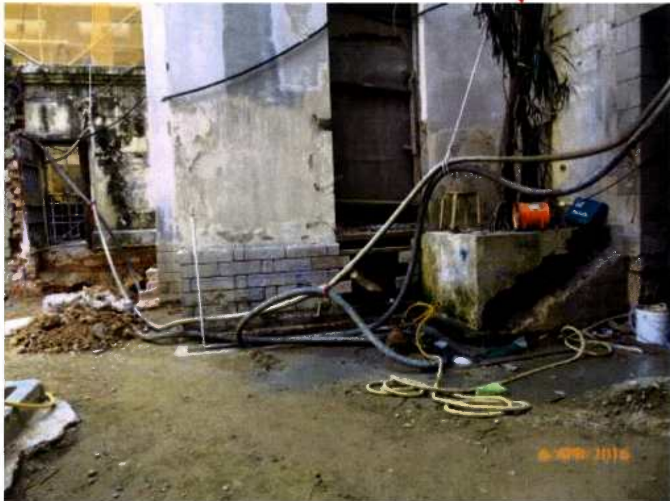
Fig. 9 Construction works are in progress near the tree .
