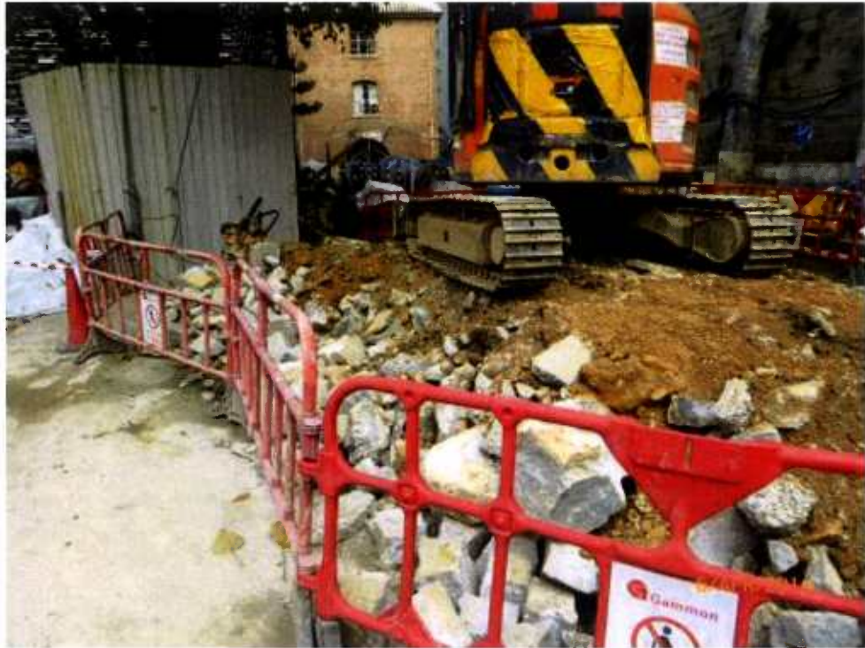
Fig. 10 Construction works are in progress near the cordon zone.
