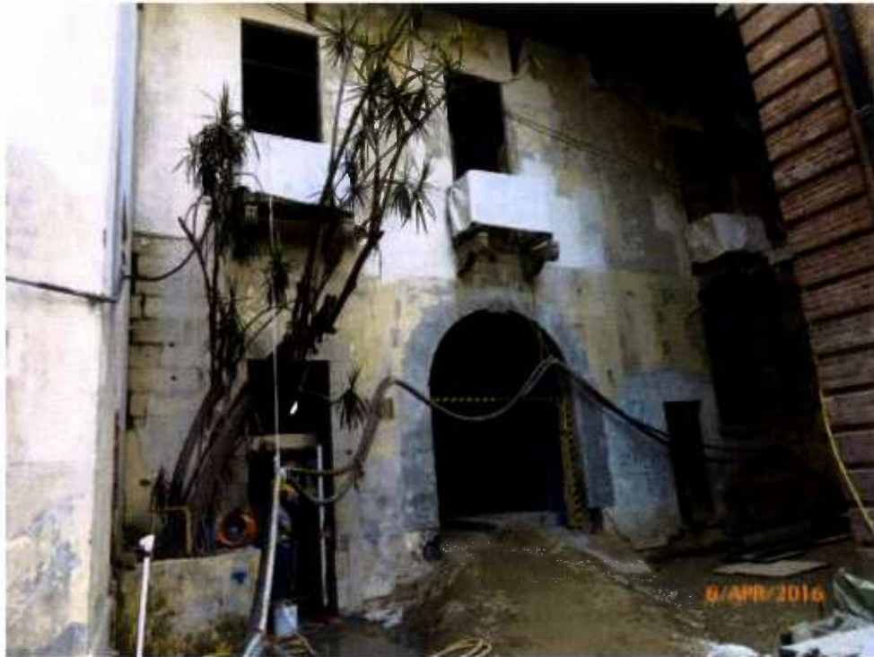
Fig. 10 The nearby buildings are under renovation.
