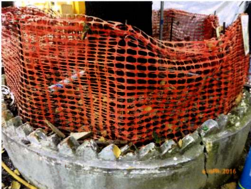
Fig. 9 The small cordon zone is in order.
