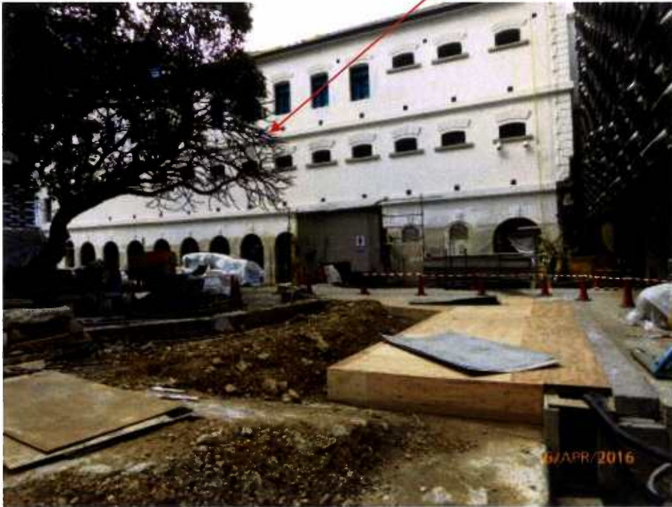
Fig. 8 Construction works are in progress near Tree 8 .
