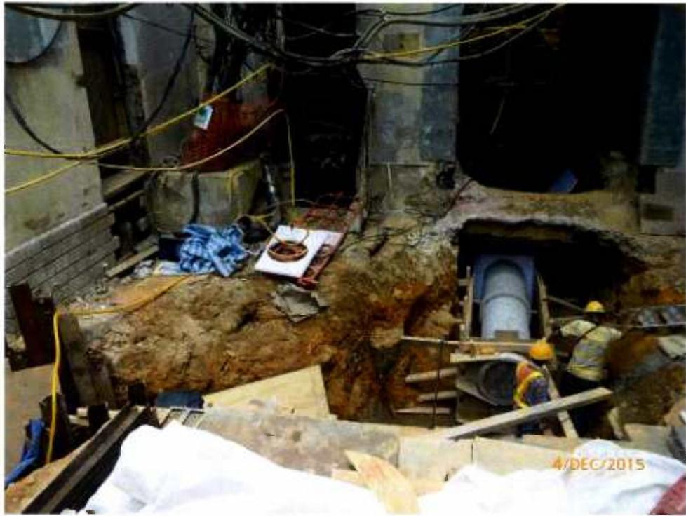
Fig. 2 The site near Tree-11 is under renovation.
