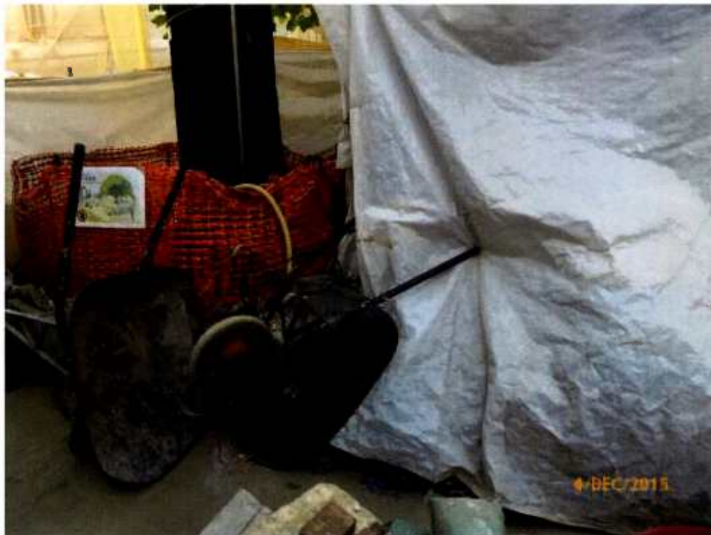
Fig. 9 Some construction instruments are placed near the planter.
