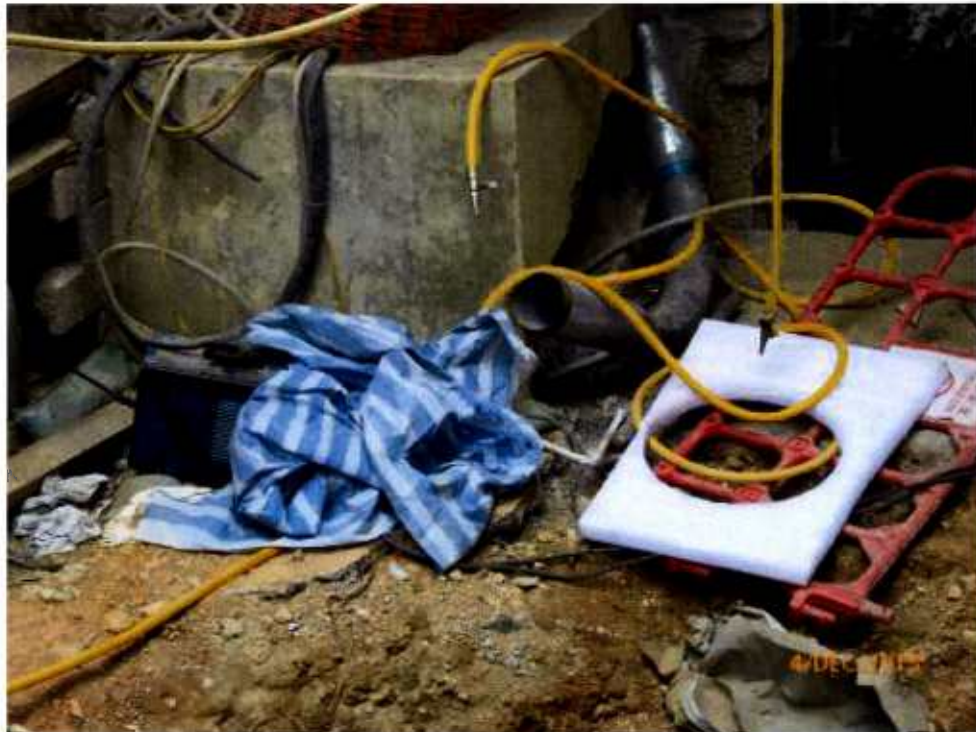
Fig. 9 Many construction materials are placed near the planter.
