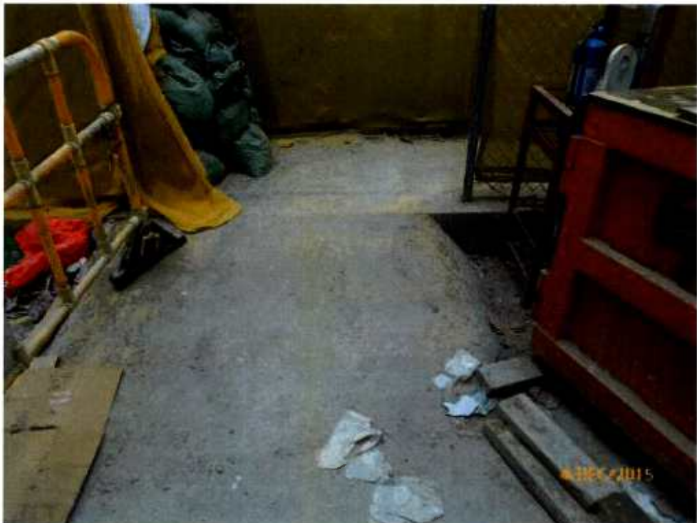
Fig. 11 Cleanliness of the access near Tree-9 is acceptable .
