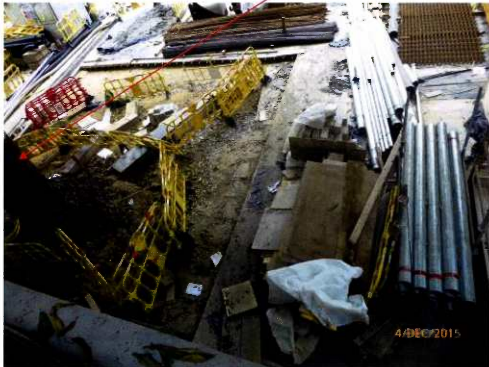
Fig. 9 Renovation work is in progress near Tree-5 .
