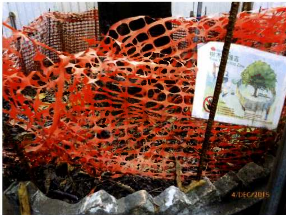
Fig. 7 The small cordon zone is in order at the planter.
