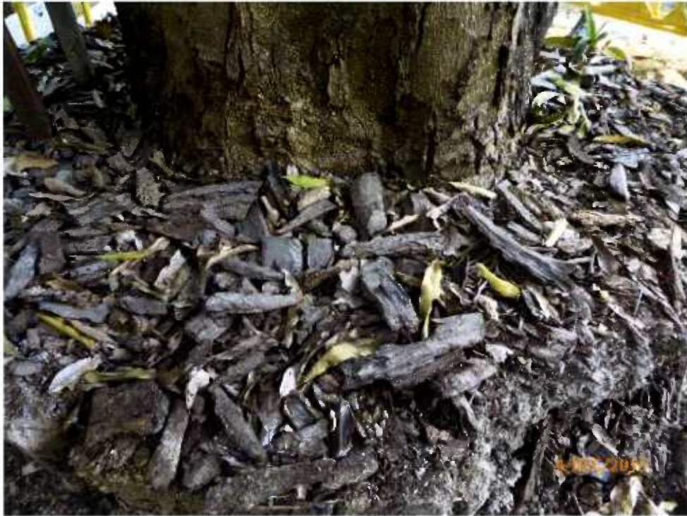
Fig. 4 Root collar is normal. The planter appears clean and tidy.
