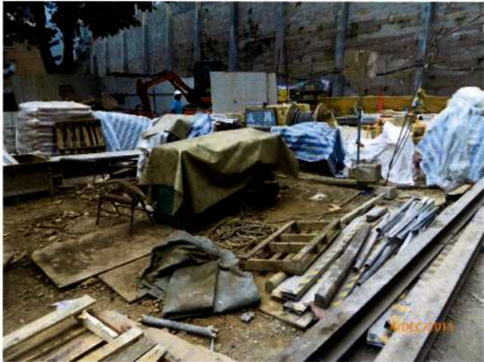
Fig. 10 Construction works are in progress near Tree-6.
