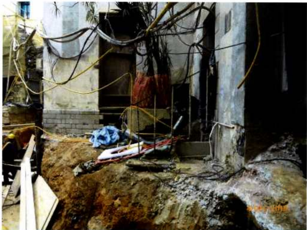
Fig. 11 The large cordon zone has been removed for renovation work.
