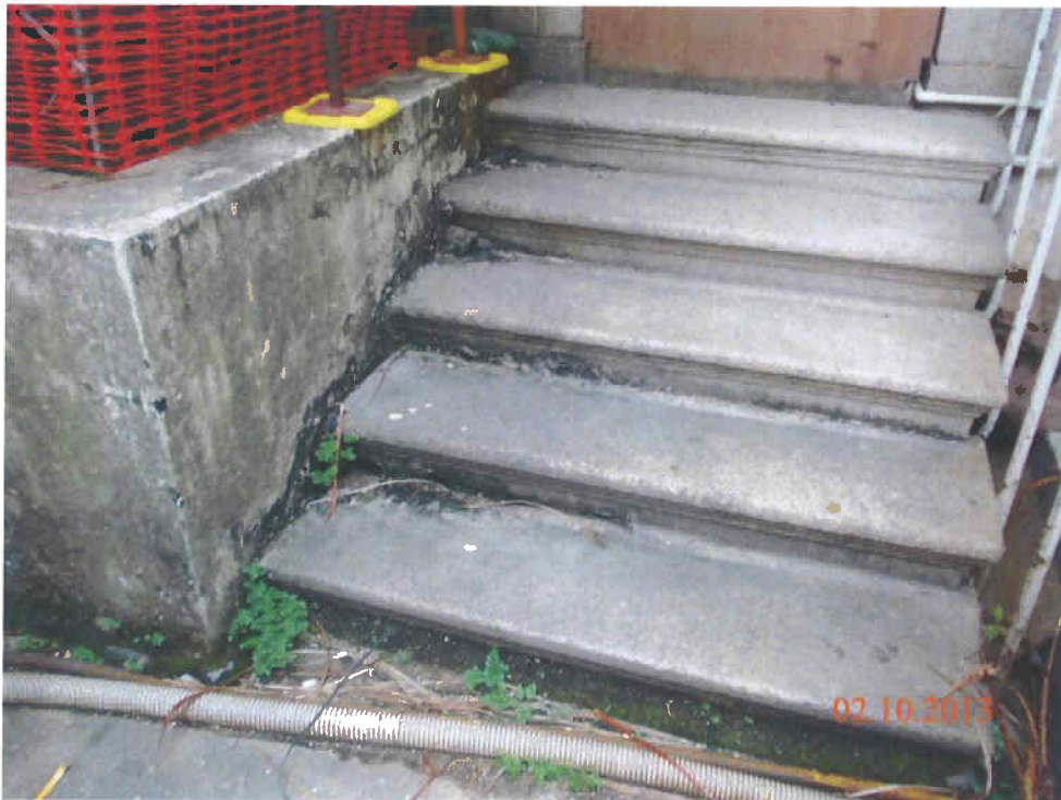
Fig. 3 Cleanliness of the site is acceptable.
