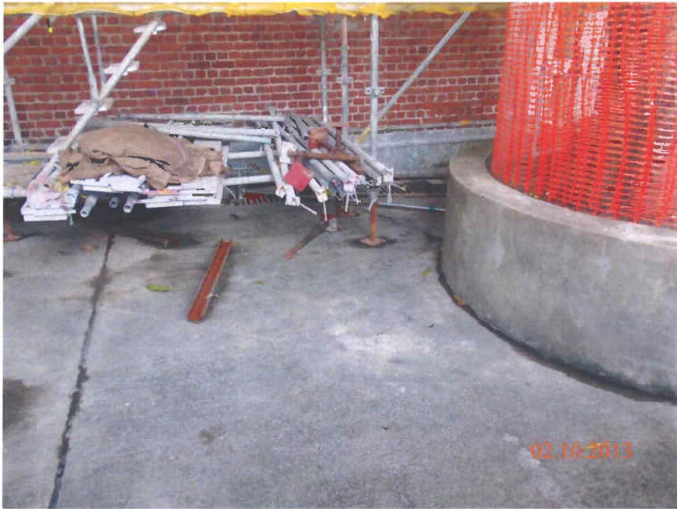
Fig. 4 The scaffold still remains at site for further renovation work.
