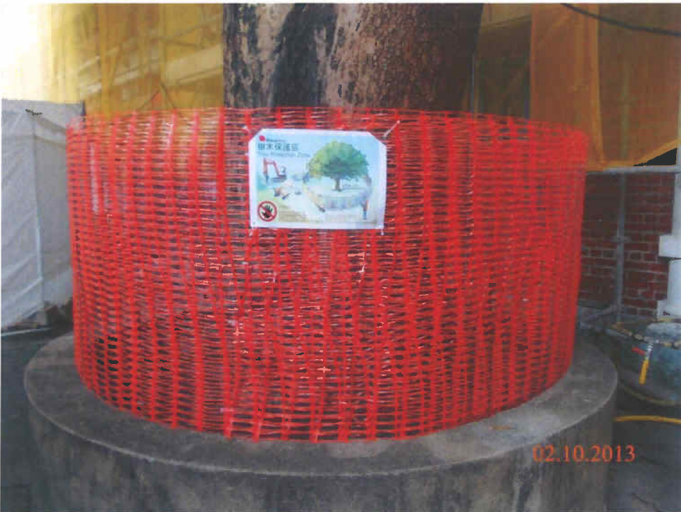
Fig. 5 A small cordon zone is newly set up to protect the tree.
