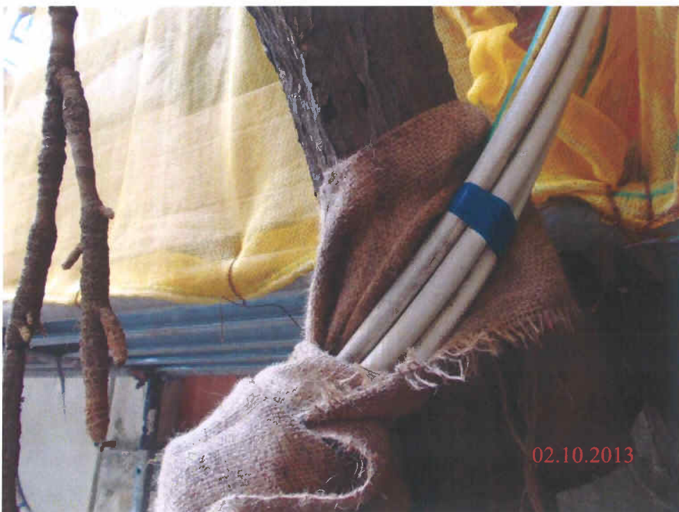
Fig. 5 The trunk has been wrapped with hessian cloth so as to get rid of damage to the tree.
