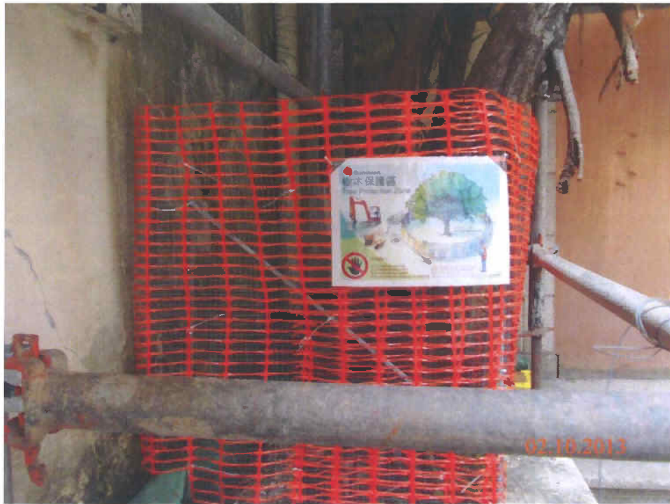
Fig. 4 A small cordon zone is newly set up to protect the tree.
