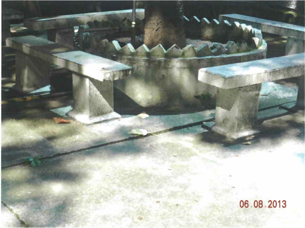
Fig 2. The planter and the site are clean and tidy at the time of inspection.
