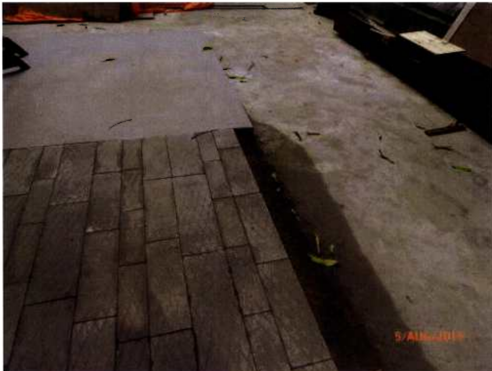
Fig. 10 The site near the entrance to Tree-5 is clean and tidy.
