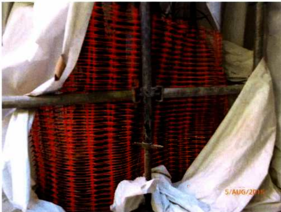
Fig. 9 The small cordon zone is in order.
