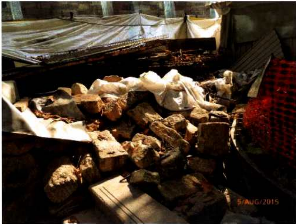
Fig. 8 Many construction items are placed near the planter.
