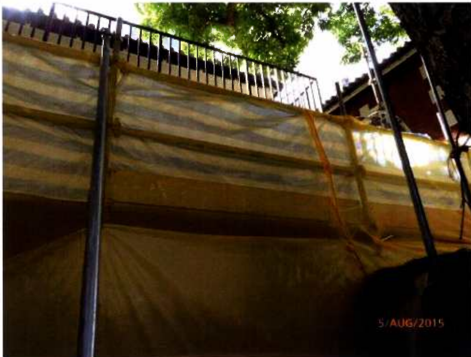
Fig. 8 Renovation works are in progress near Tree-5.
