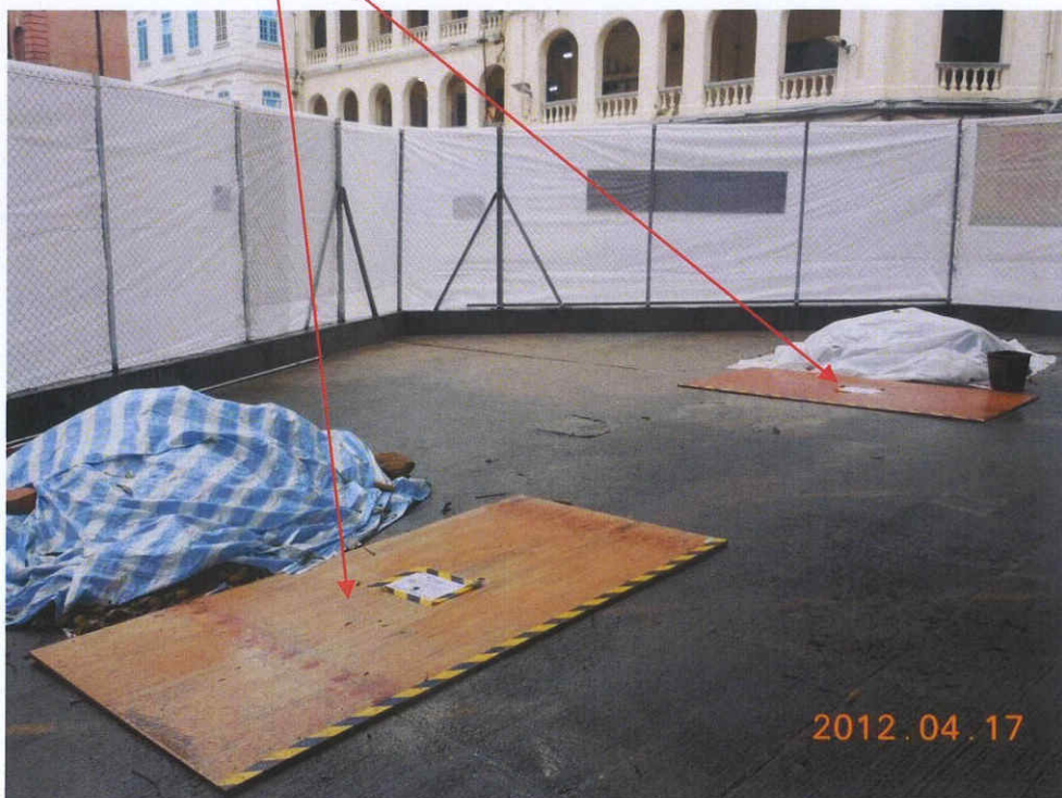
Fig. 5 Two trial pits have been excavated inside the cordon zone.
