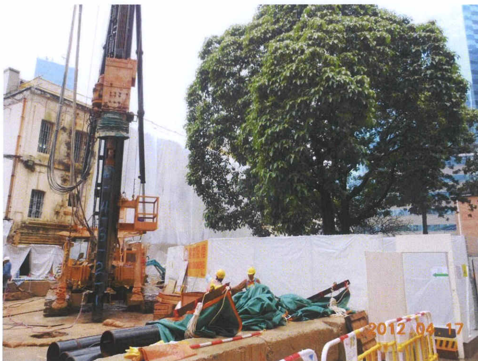
Fig. 5 Construction works commence near the cordon zone.
