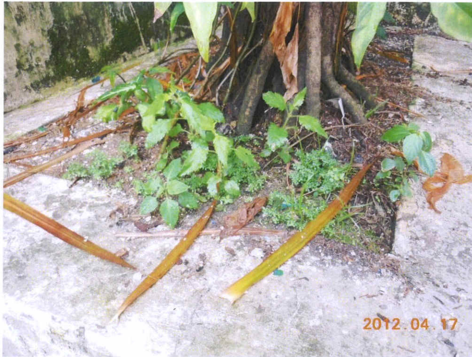
Fig. 2 Condition of the planter is acceptable at the time of inspection.
