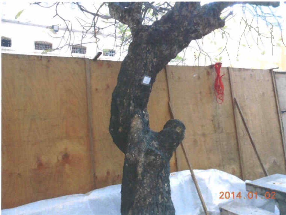
Fig. 5 Health condition of the main trunk is fair.
