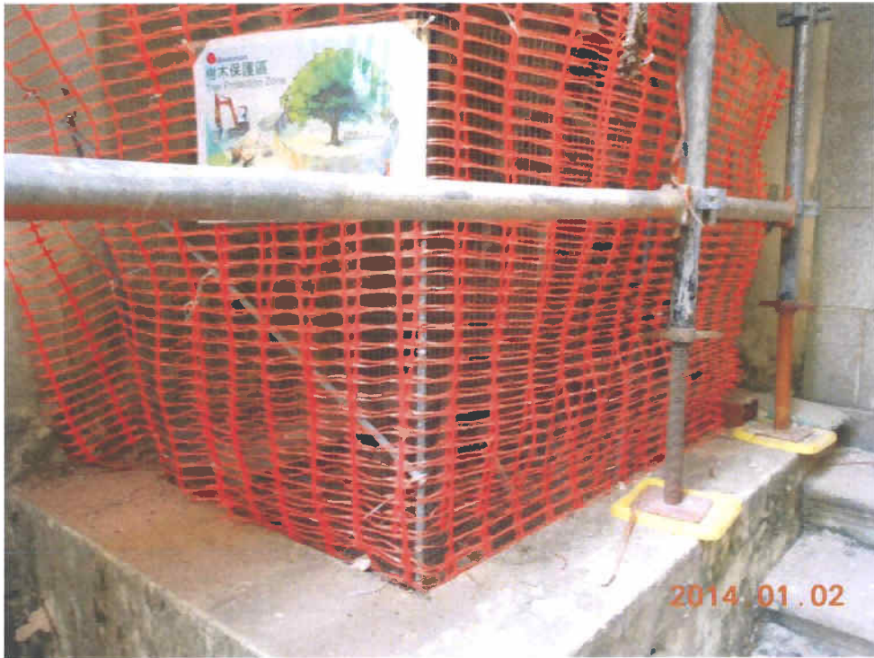
Fig. 4 A small cordon zone is set up to protect the tree.
