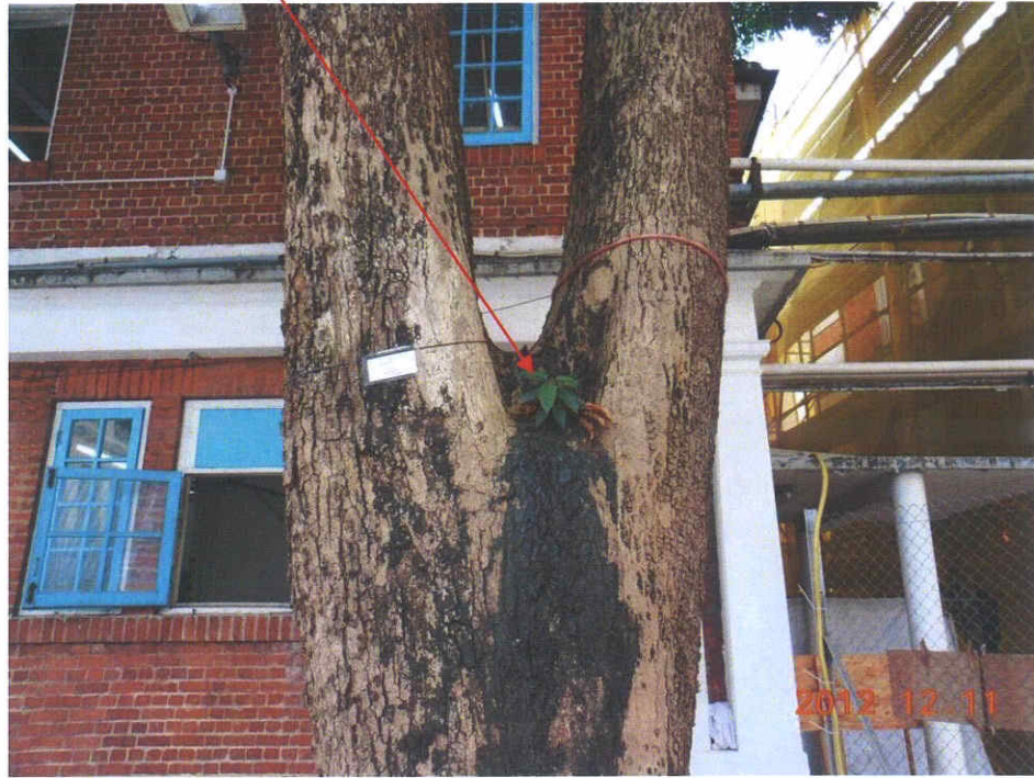
Fig. 4 Parasitic plant appeared on Tree-5 during inspection on 11.12.2012.
