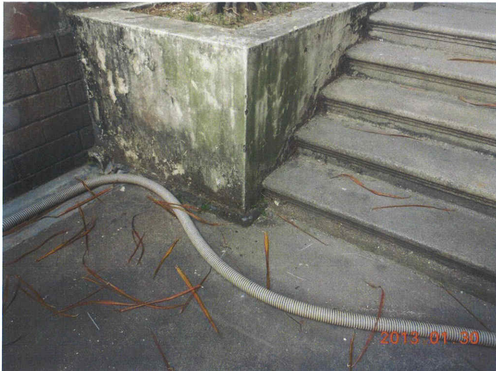
Fig. 3 Cleanliness of the site is acceptable.
