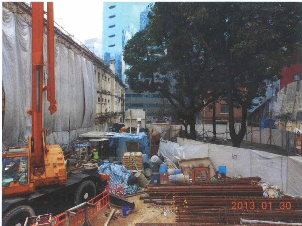
Fig. 5 Construction works in progress outside the cordon zone.
