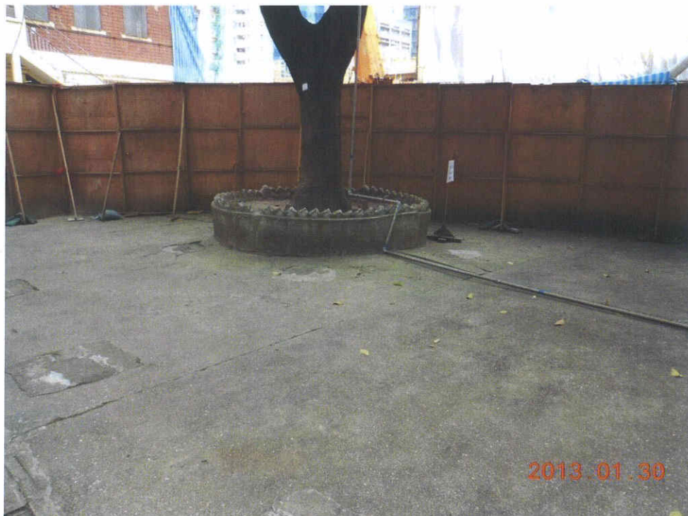
Fig. 5 The site appears clean and tidy on 30.1.2013.
