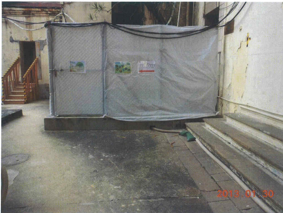
Fig. 5 The site outside the cordon zone is clean and tidy.
