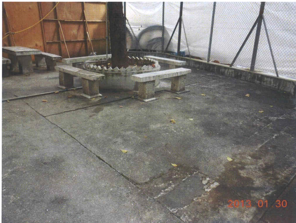
Fig. 4 The site appears clean and tidy at the time of inspection.
