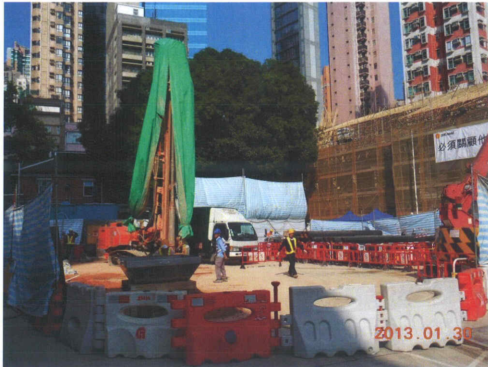
Fig. 6 Construction works in progress near the cordon zone
