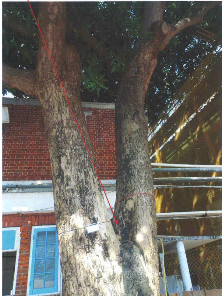
Fig. 5 The plant has been removed prior to inspection on 30.1.2013.
