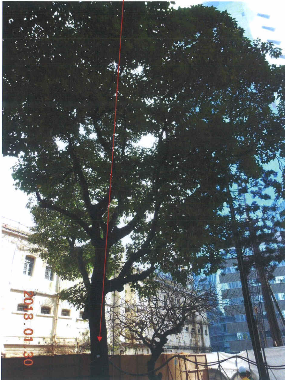
Fig. 6 Overall view of Tree-7 during inspection on 30.1.2013.
