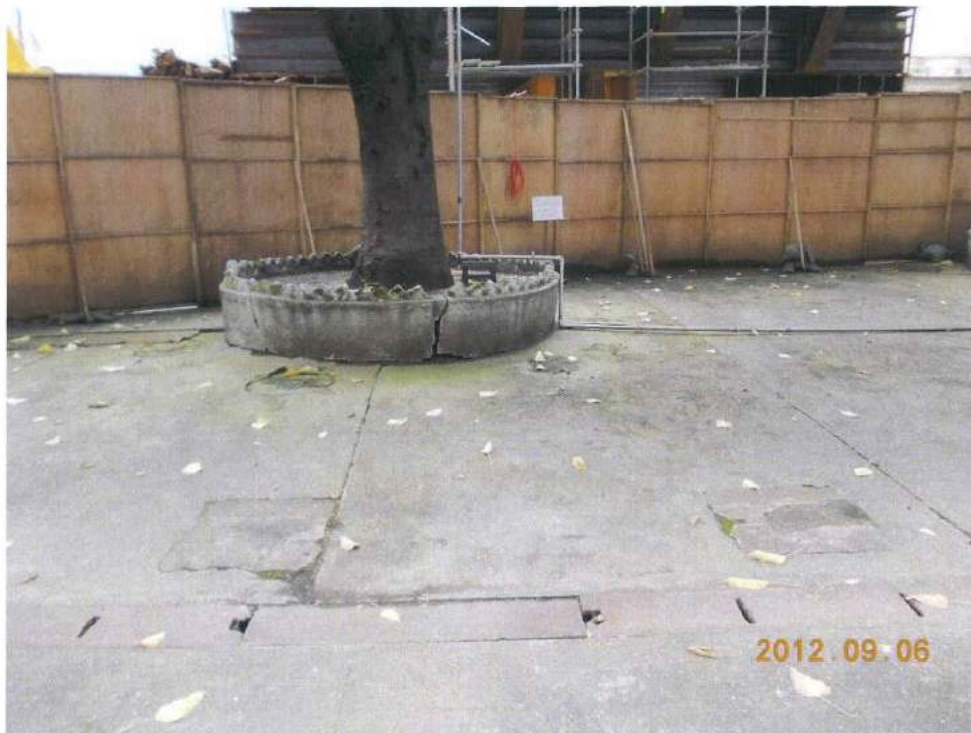
Fig. 5 Cleanliness of the site is acceptable.
