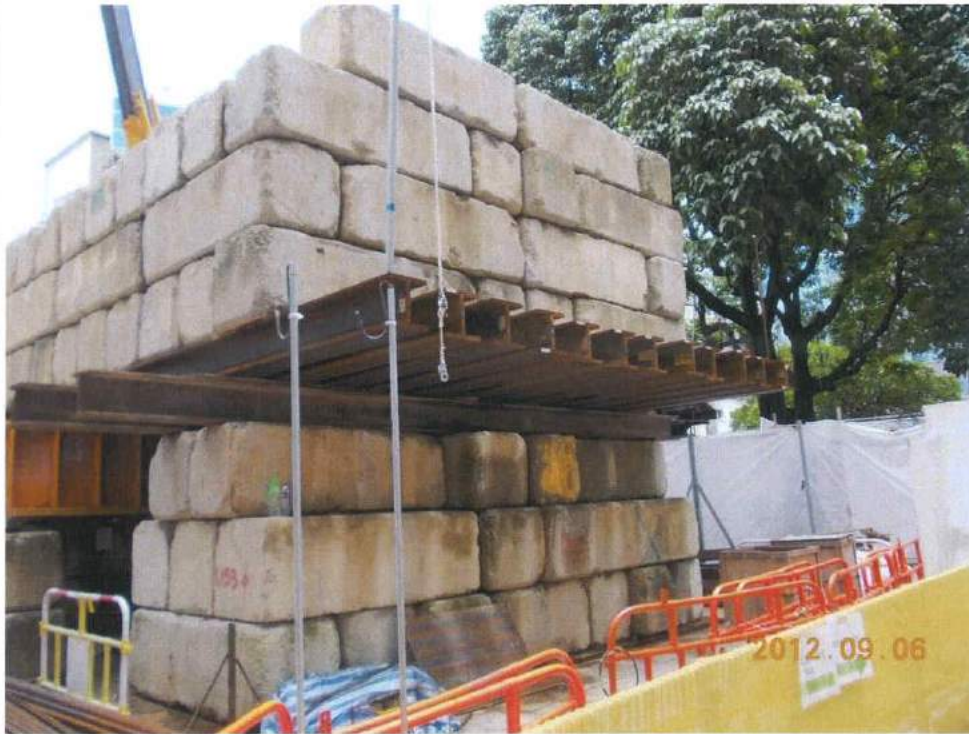
Fig. 6 Lots of bulky item are placed outside the cordon zone.
