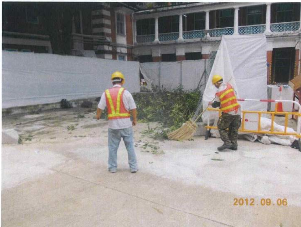
Fig. 7 Skilled workers tidy up the site after trimming work.
