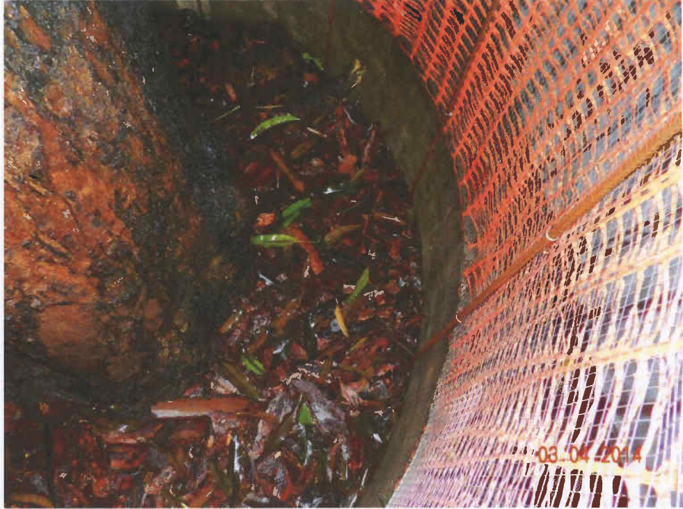
Fig 2. Root collar of Tree-5 is good. Sufficient mulch has been added at the planter.
