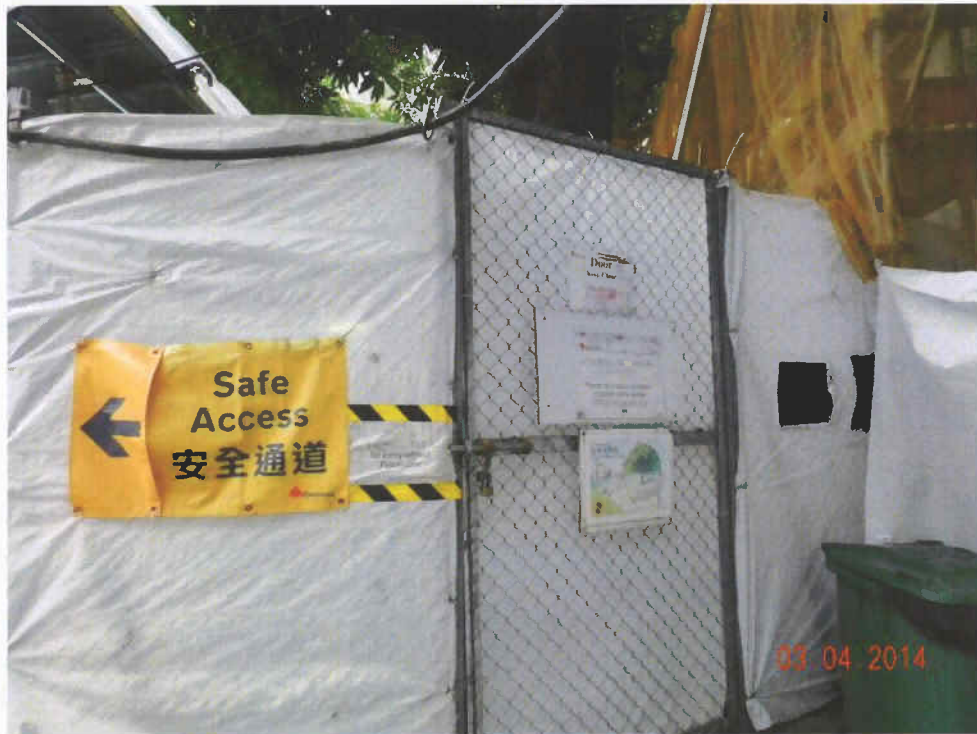
Fig. 9 The door is locked up prior to inspection.
