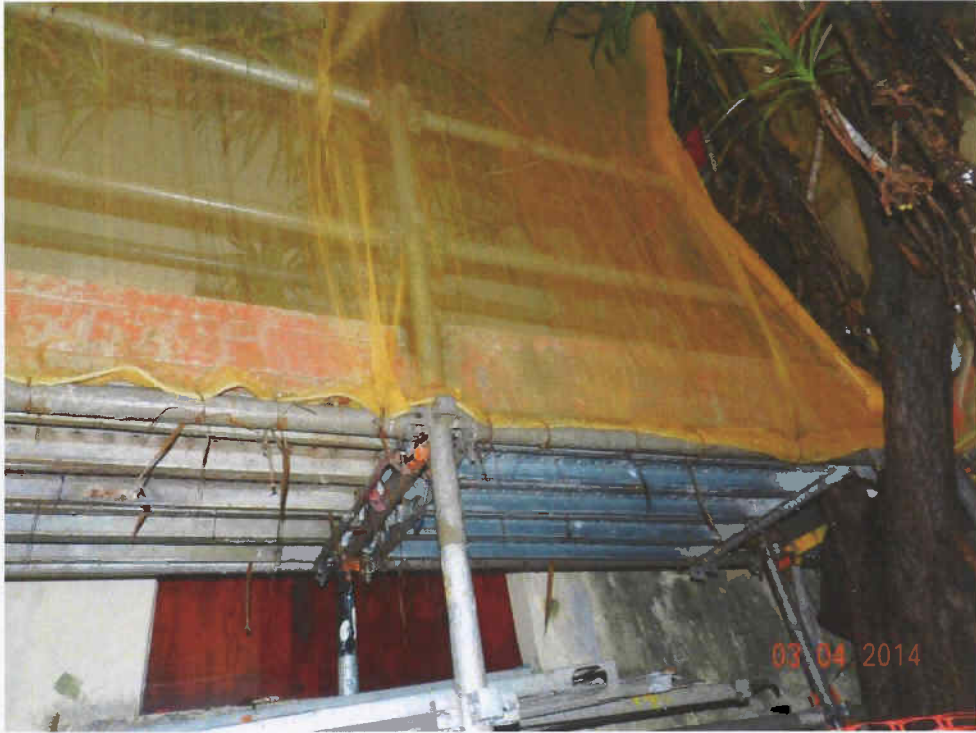
Fig. 4 Renovation works are in progress near the tree.
