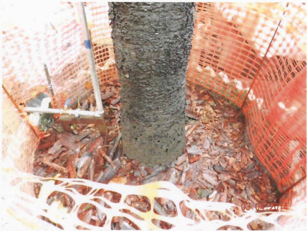
Fig 2. Root collar of Tree-9 is normal. Sufficient mulch has been added at the planter.
