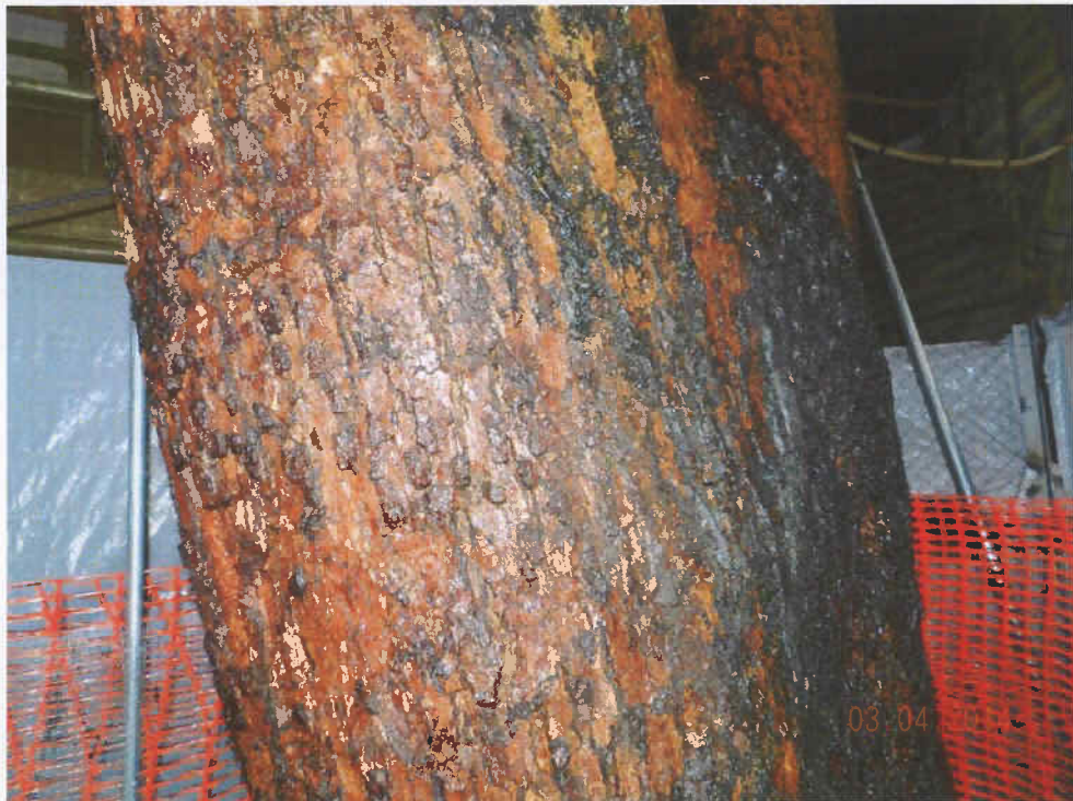
Fig. 3 Health condition of the mid trunk is good.
