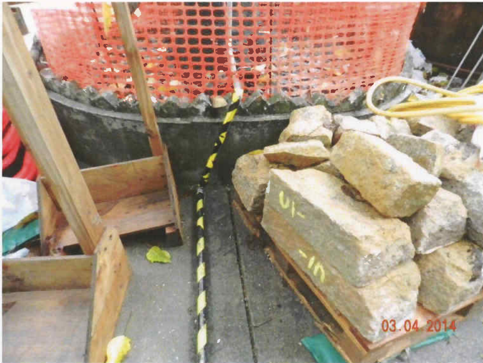
Fig. 6 Bulky items are placed near the planter but cause no disturbance to the tree.
