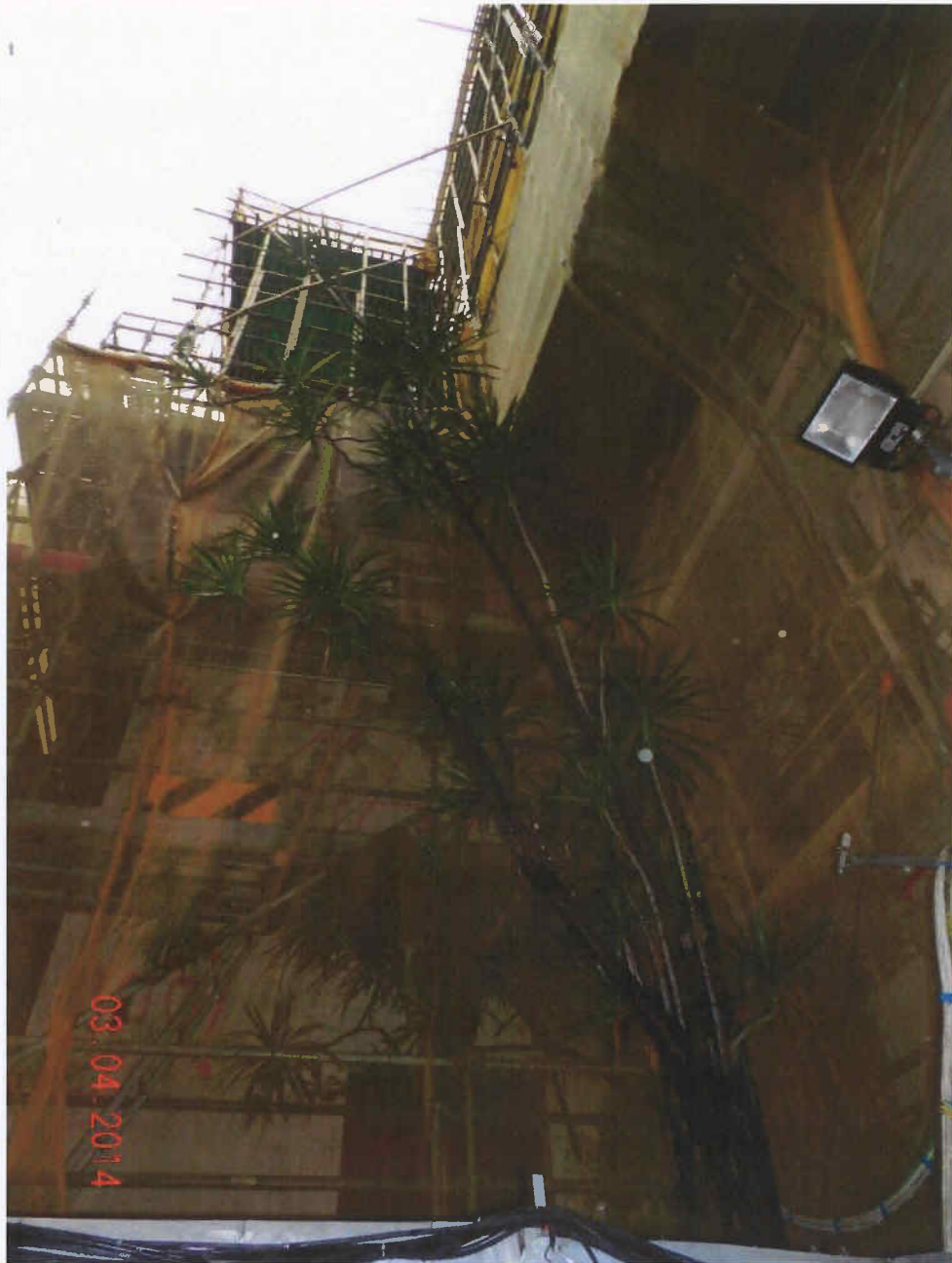
Fig. 8 Overall view of Tree-11 during inspection on 3 rd April 2014.
