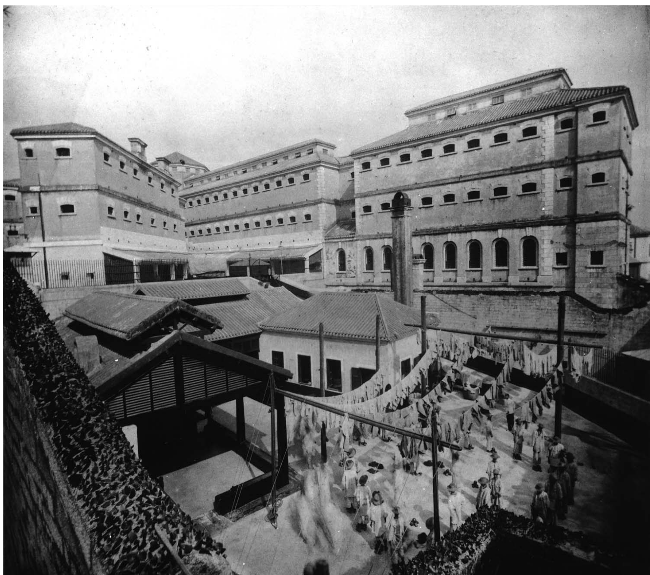
Figure 3.3 View looking into the Victoria Gaol radial plan prison c.1895, showing the laundry yard area and D Hall
