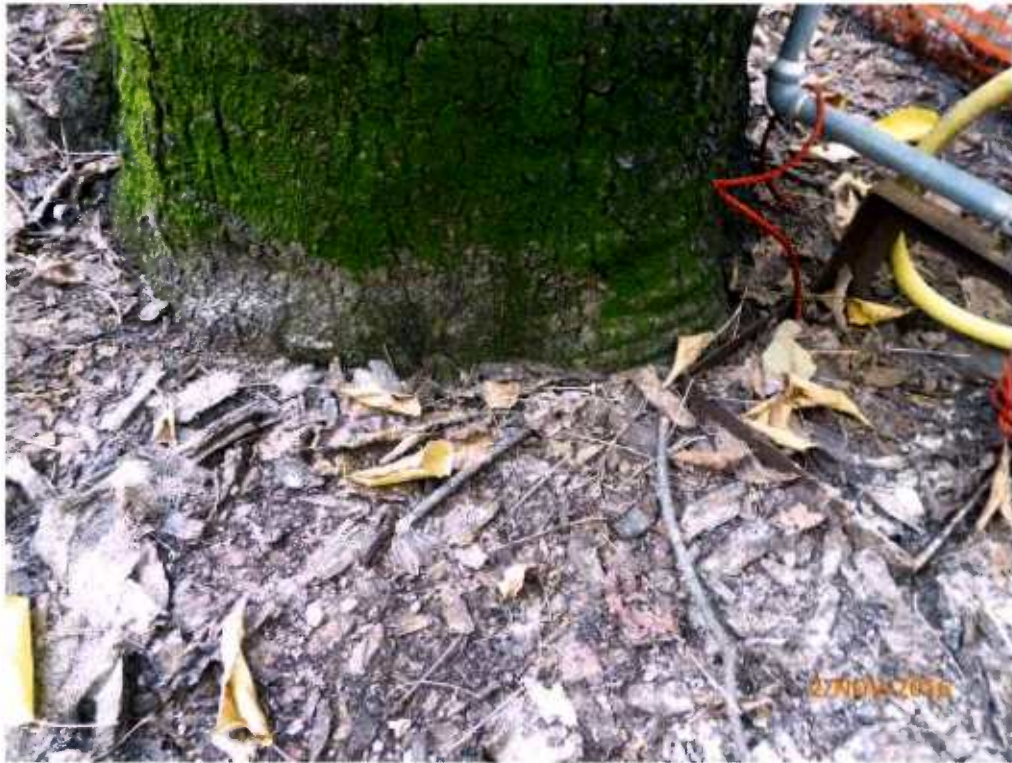
Fig 2. Root collar is normal. The topsoil is covered with mulch and leaves.
