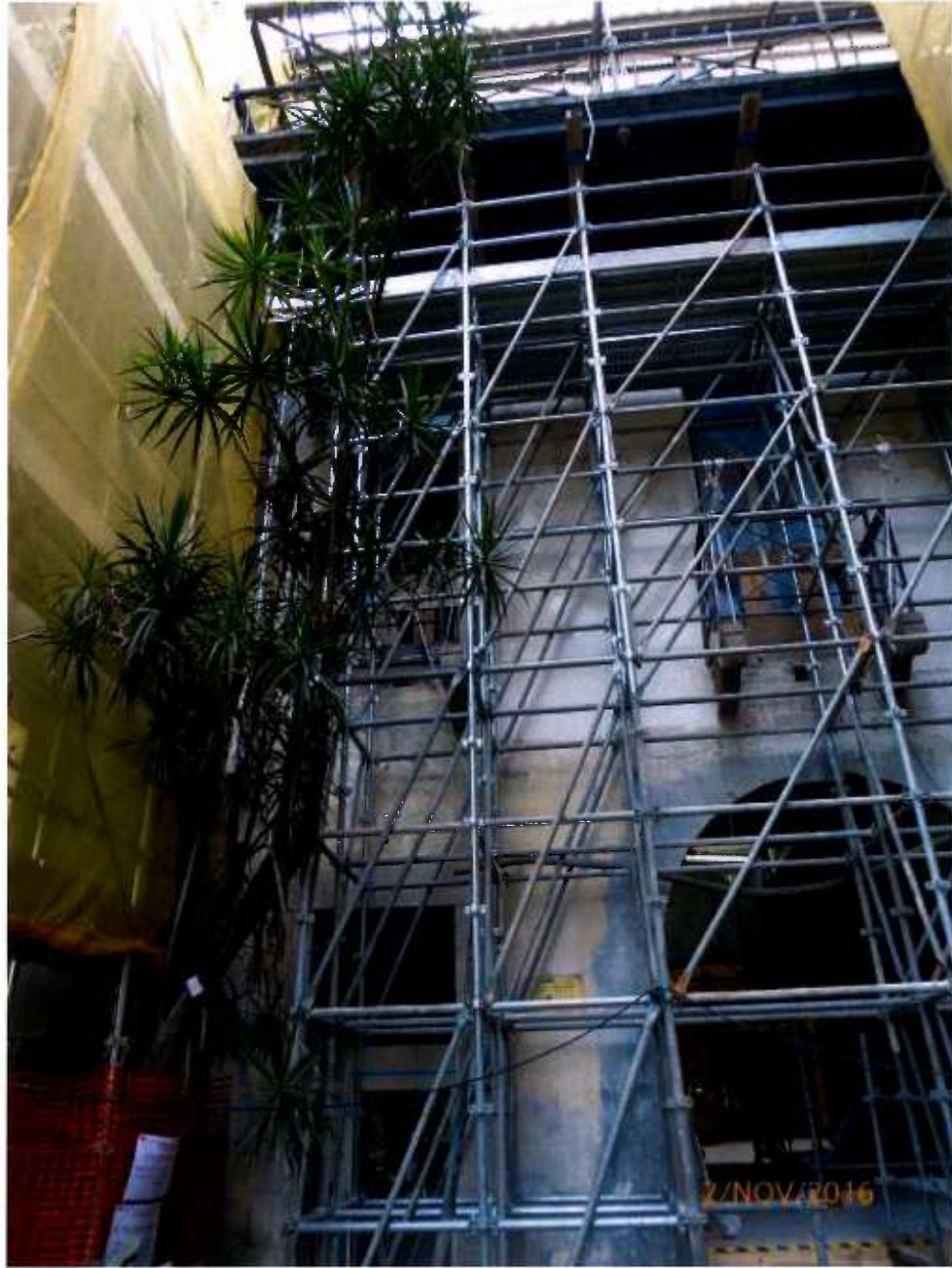
Fig. 12 Overall view of Tree-11 during inspection on 2 nd November 2016.
