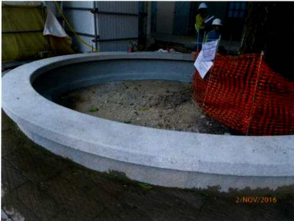
Fig. 10 The newly-built planter still vacated and pending for backfilling of topsoil.
