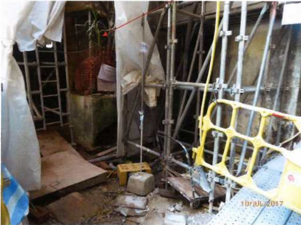
Fig. 11 Renovation works are in progress near Tree-11 .
