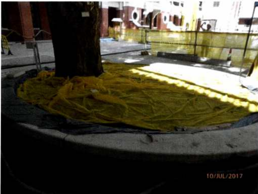
Fig. 9 The newly-built planter is covered with some netting sheets.
