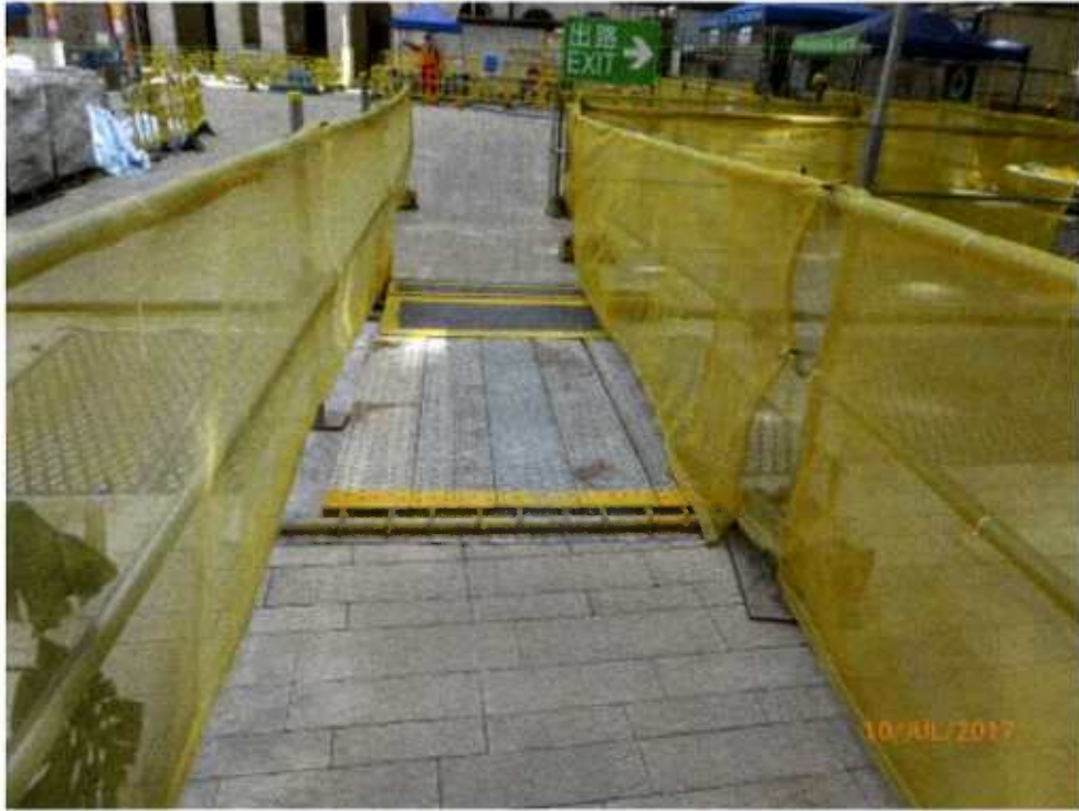
Fig. 10 The access near the planter is clean and tidy.
