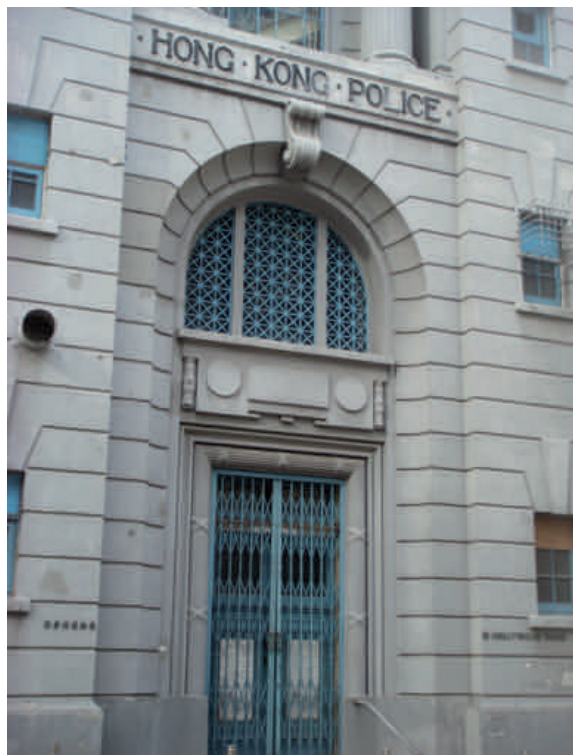
Detail of the Headquarters Block north entrance. Note the architectural features similar to those of the Fringe Club.
