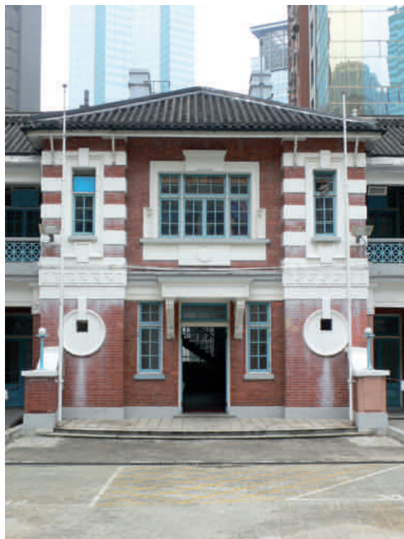
View of the central bay of the Headquarters Block showing brick and render similar to the Fringe Club.
