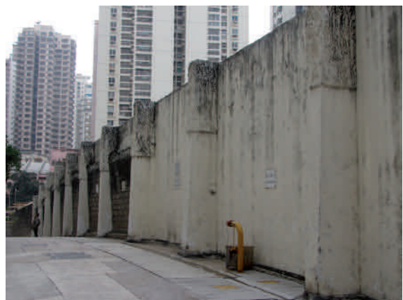
The security wall on Chancery Lane
