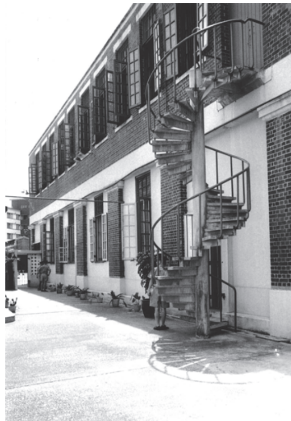
F Hall exterior
