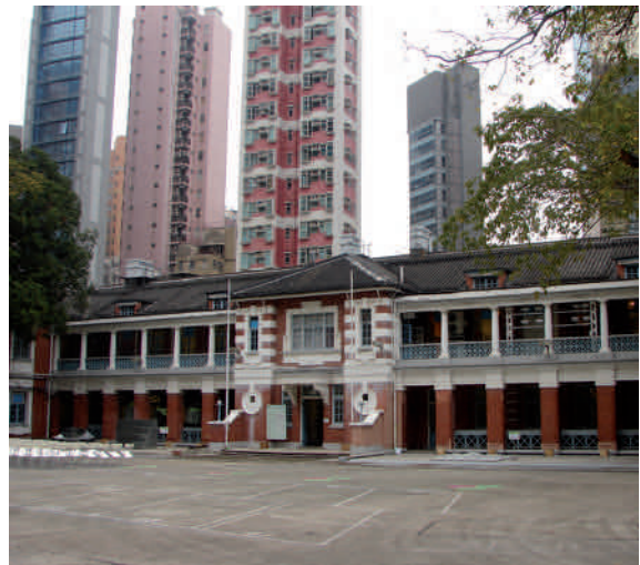
View of the south façade of the Headquarters Block facing the Parade Ground
