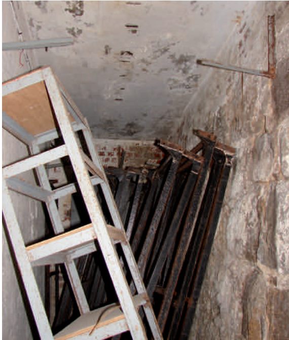
Ladder store with blocked archway
