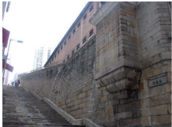
The historic steps on Chancery Lane
