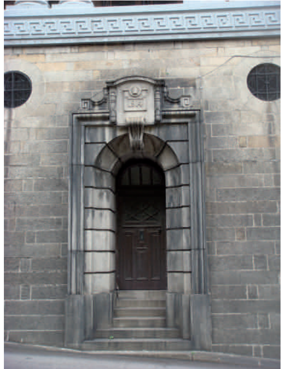
East Magistracy door at street level on Arbuthnot Road
