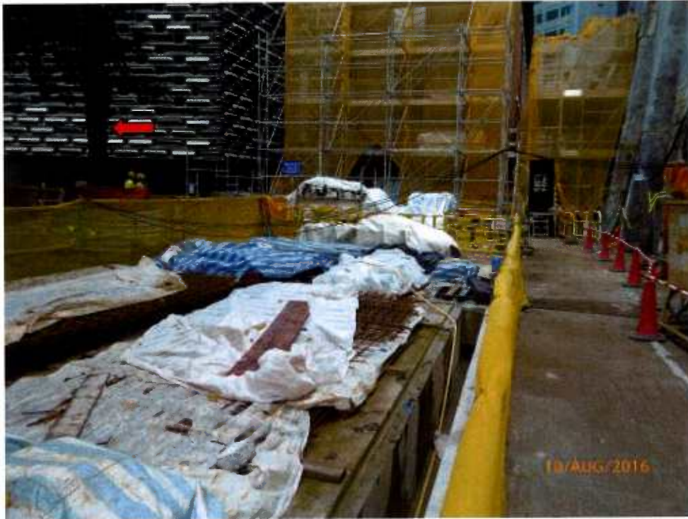
Fig. 10 Construction works are in progress near Tree-9.
