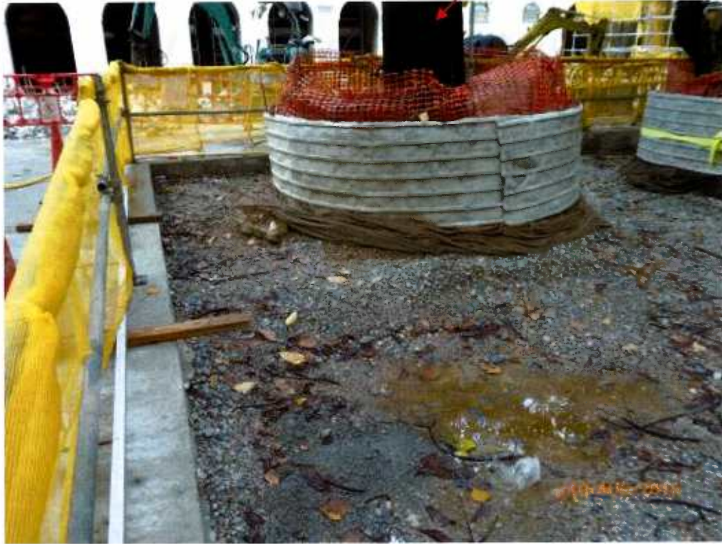
Fig. 10 Renovation works are in progress near Tree-7 .
