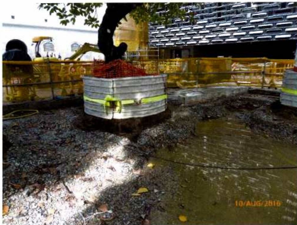
Fig. 9 The site near Tree-8 is under renovation.
