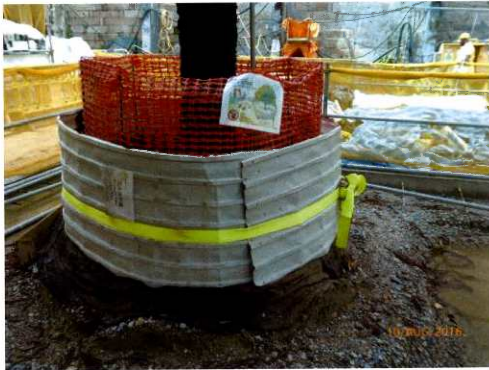
Fig. 8 Small cordon zone is in good order.
