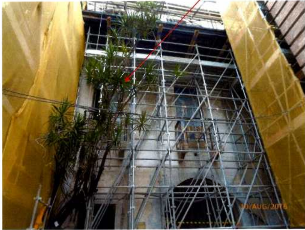
Fig. 10 Renovation works are in progress near Tree-11 .
