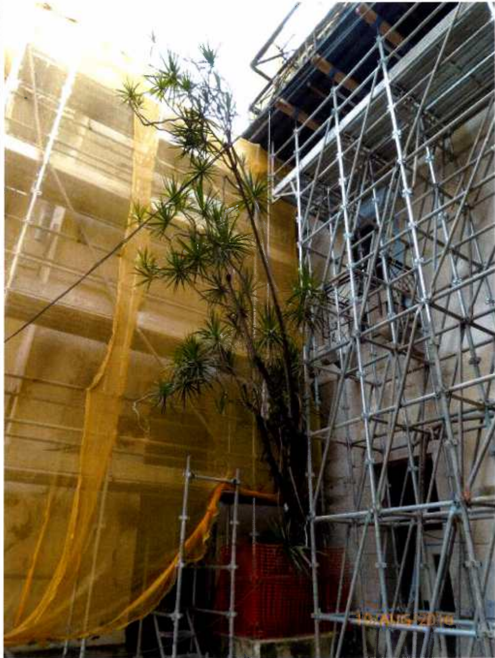
Fig. 12 Overall view of Tree-11 during inspection on 10 th August 2016.
