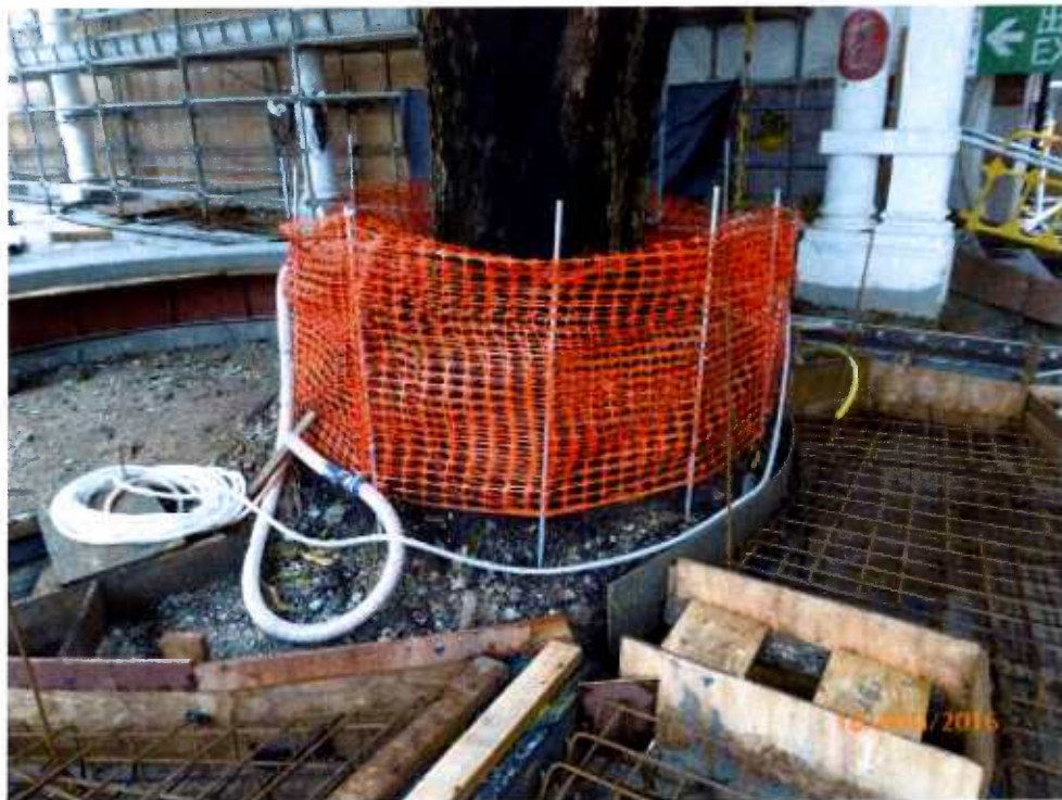
Fig. 9 The newly-erected small cordon zone is in good order.
