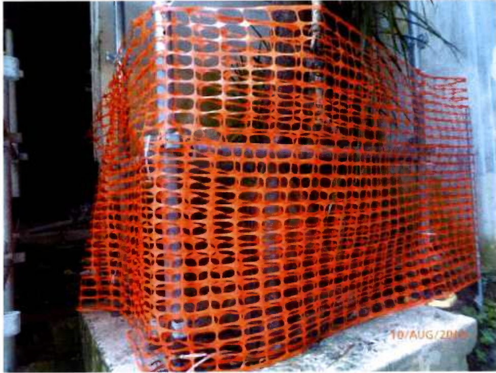
Fig. 8 The newly-erected small cordon zone is in good order.
