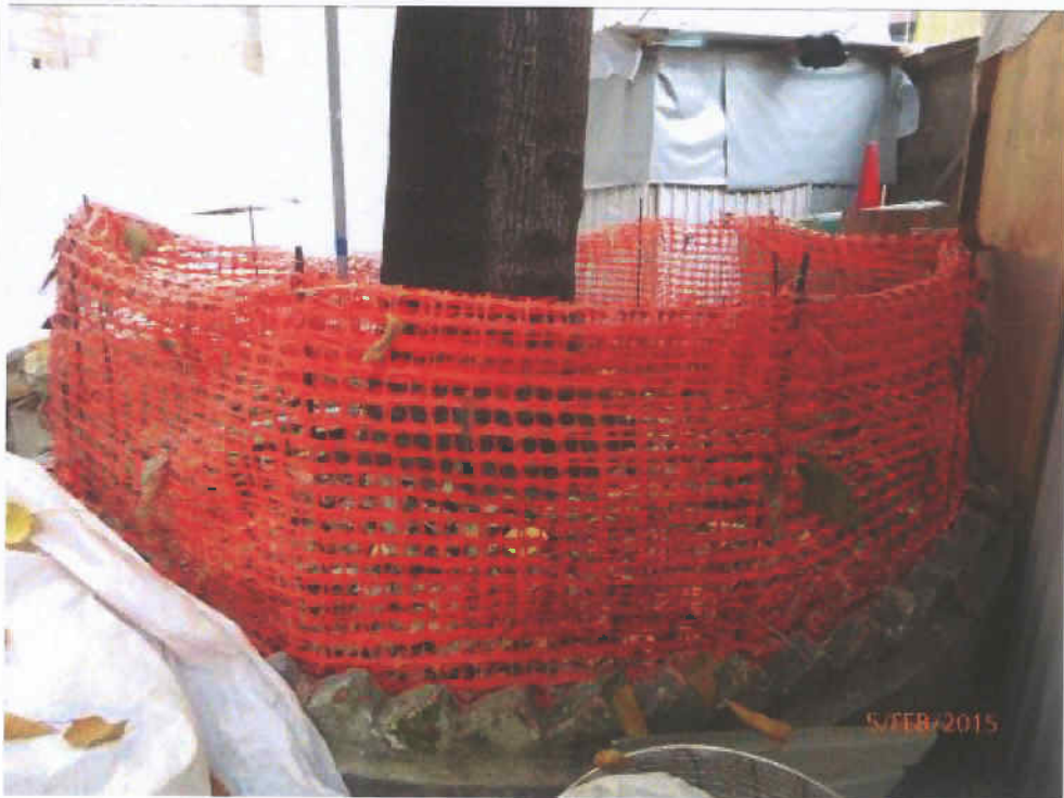
Fig. 7 The small cordon zone is in order.
