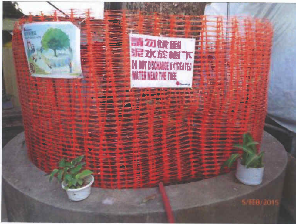
Fig. 8 The small cordon zone is in good order.
