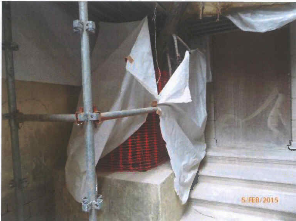
Fig. 9 The small cordon zone is in order.
