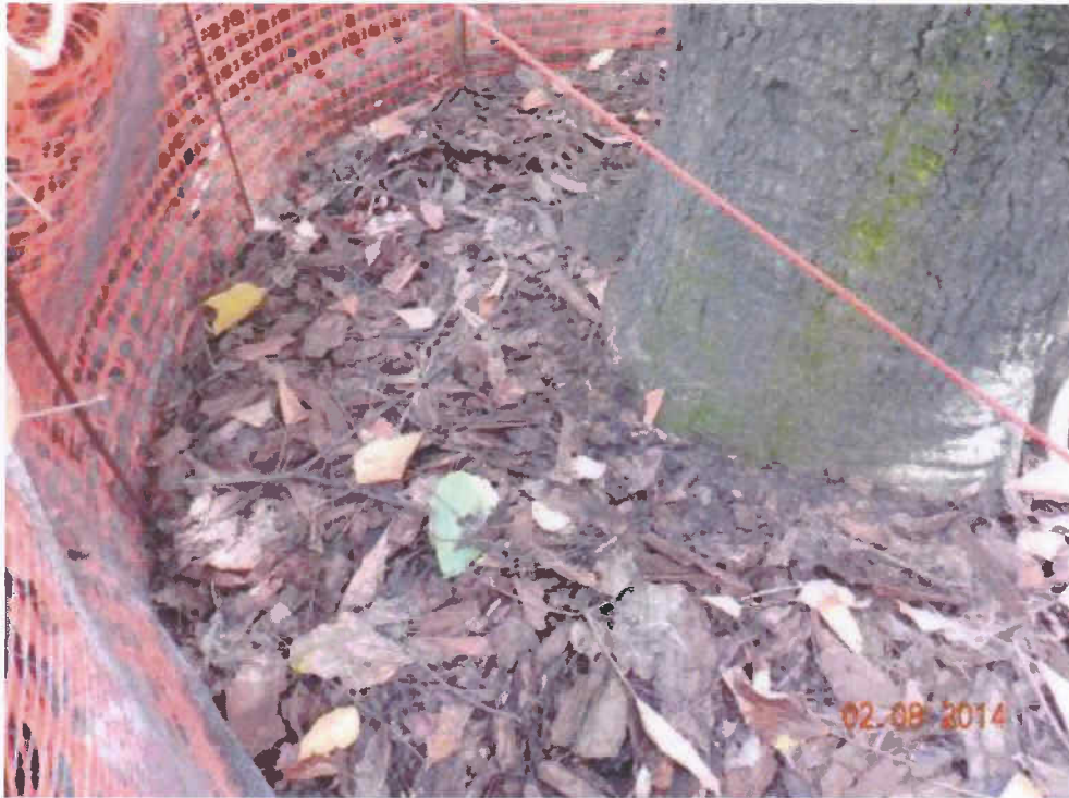
Fig 2. Root collar of Tree-7 is normal. The planter is full of mulch.
