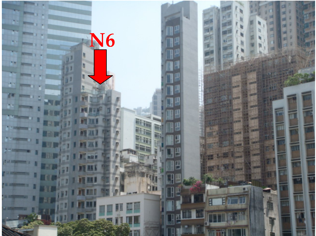
Alternative Baseline Noise Monitoring Station (N6)
