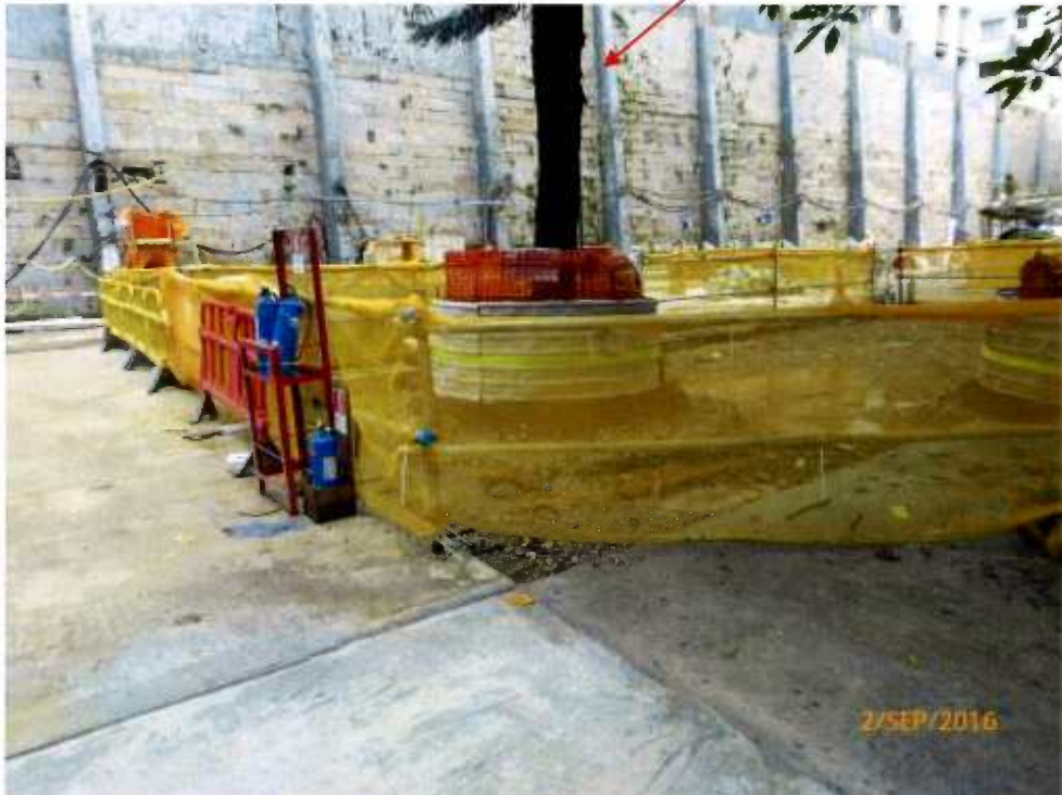
Fig. 9 A large cordon zone is newly set up near Tree-9 .
