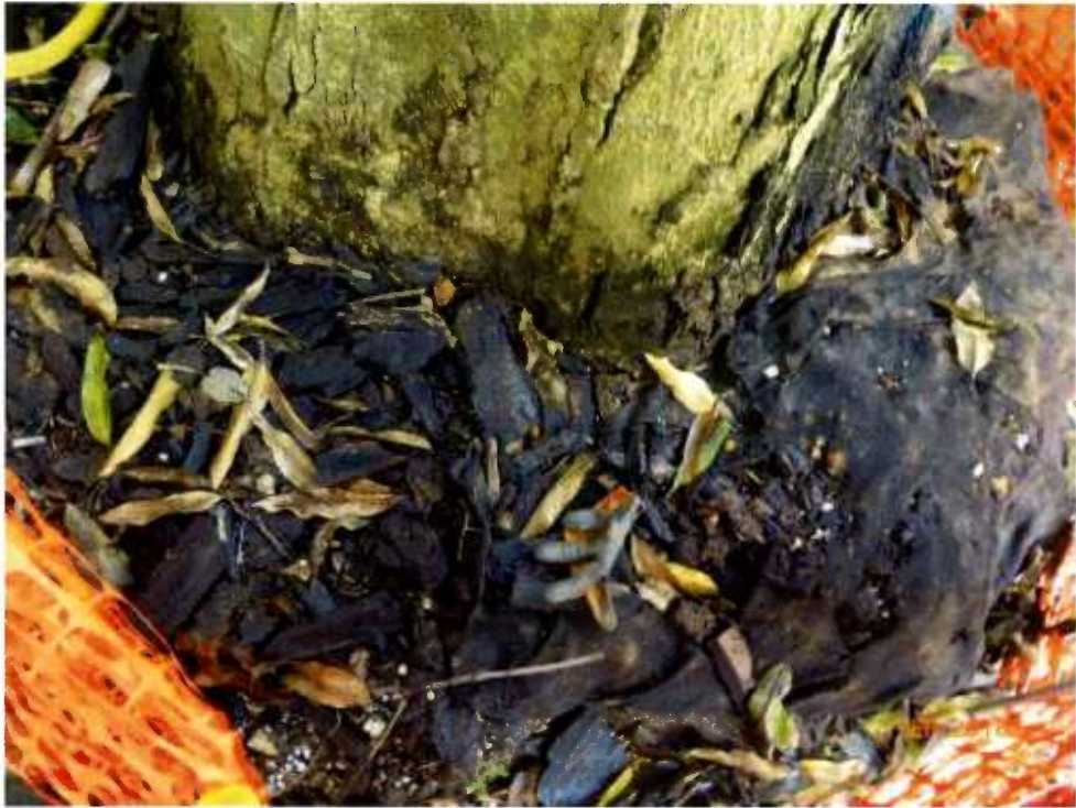
Fig 2. Root collar is normal. The planter is covered with mulch and leaves.
