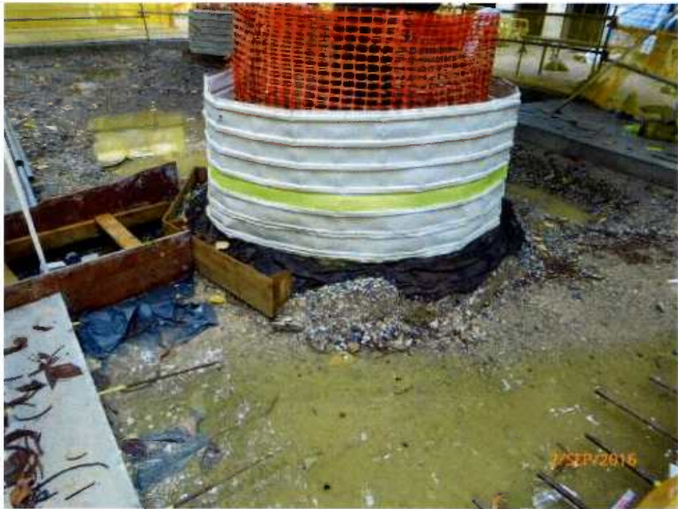
Fig. 8 Renovation works are in progress near the tree.
