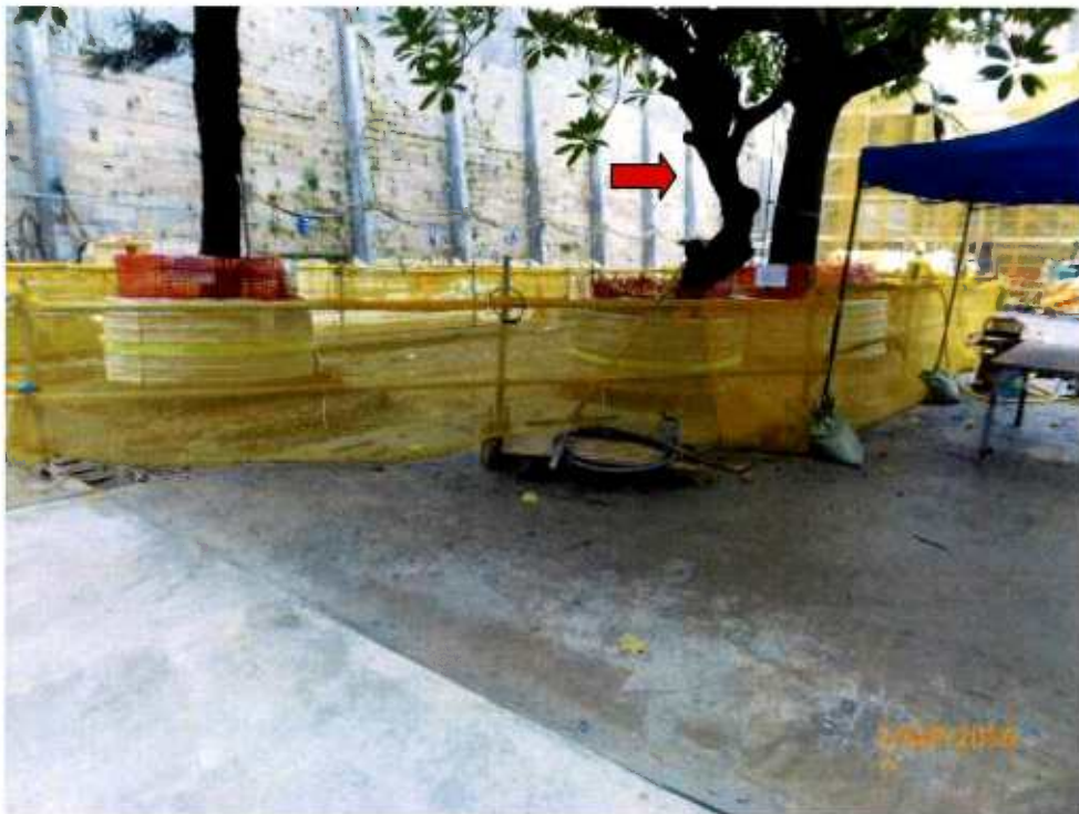
Fig. 11 A large cordon zone is newly set up near Tree-8.
