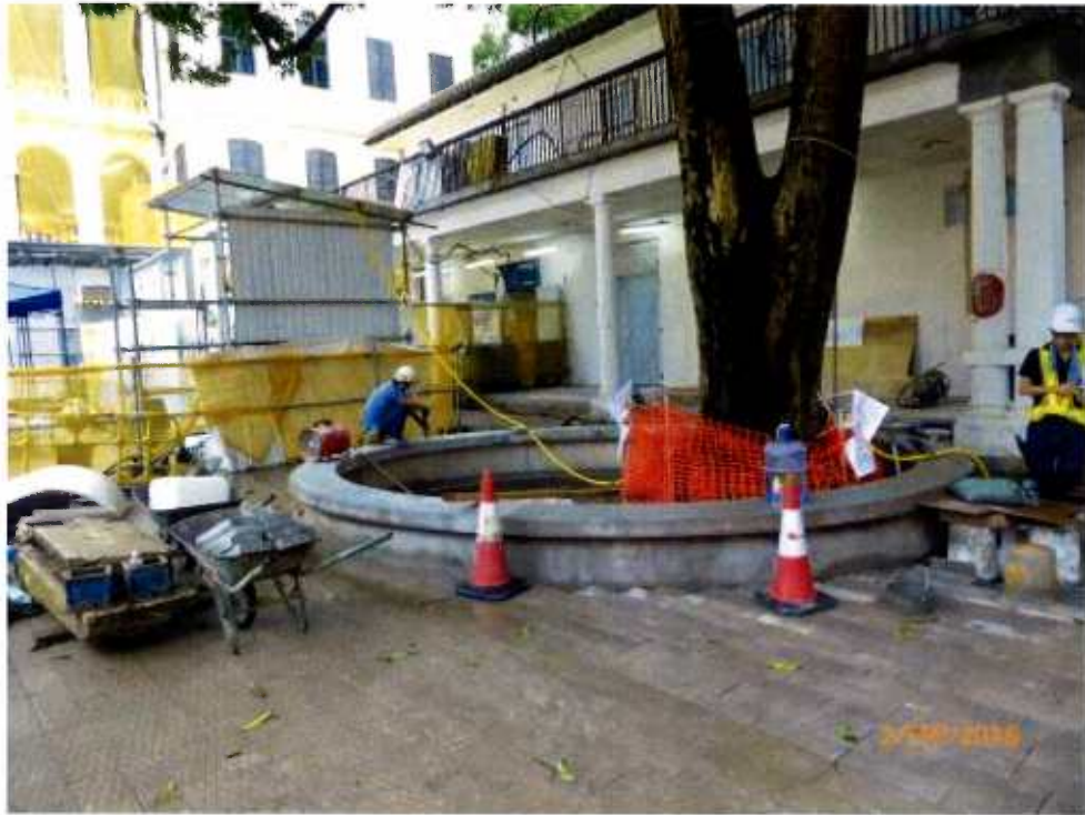
Fig. 10 A large planter is being built to replace the old one.
