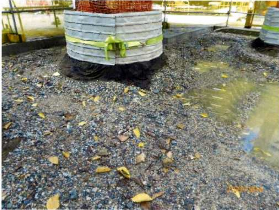
Fig. 10 Renovation works are in progress near the tree.
