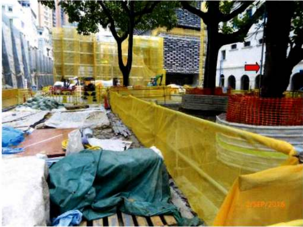
Fig. 10 Construction works are in progress outside the large cordon zone.
