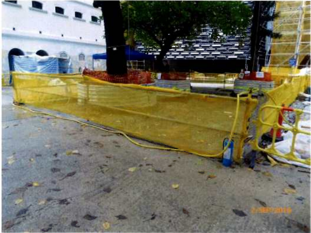
Fig. 12 A large cordon zone is newly set up near Tree-7.
