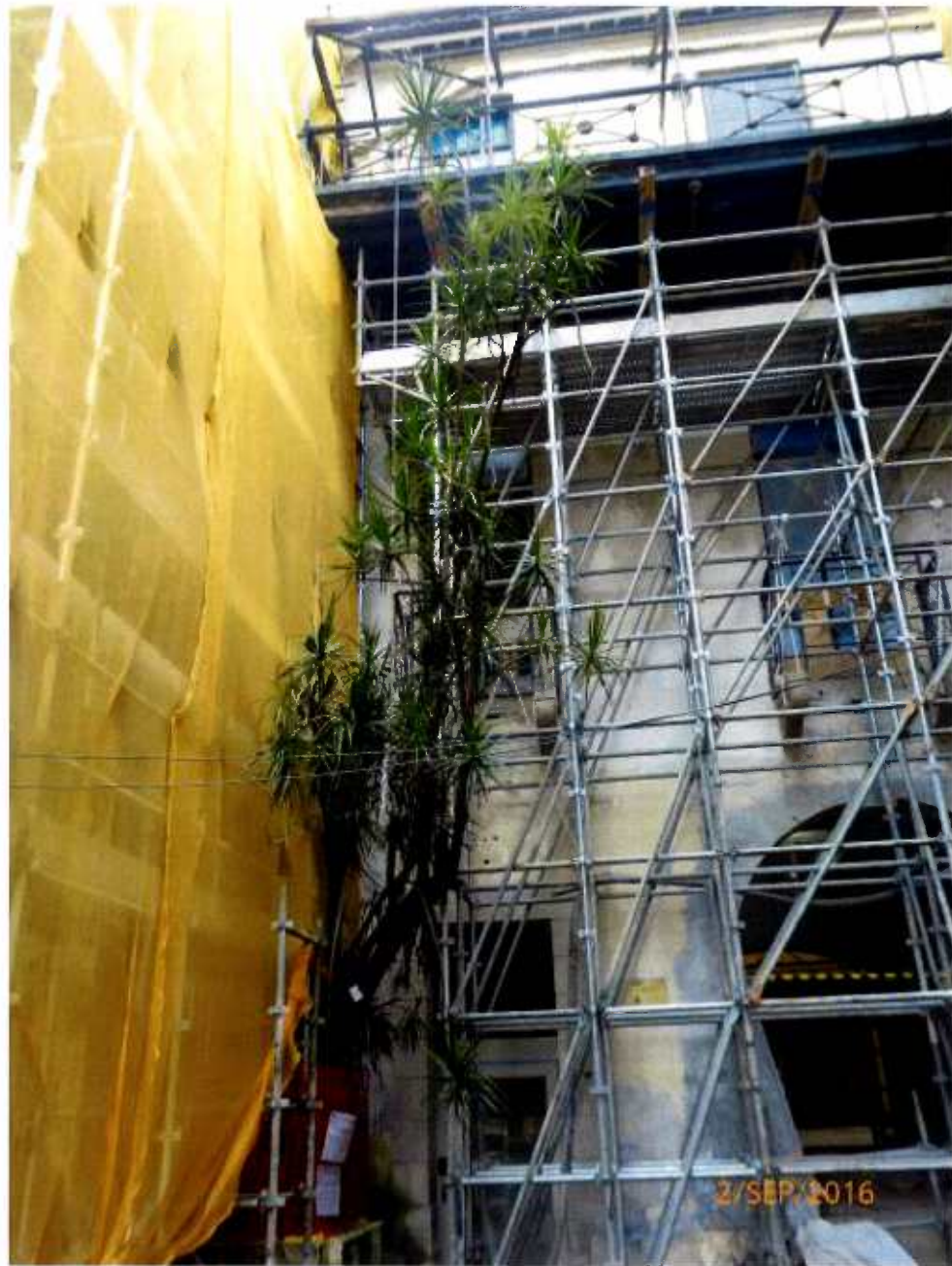
Fig. 12 Overall view of Tree-11 during inspection on 2 nd Sept. 2016.
