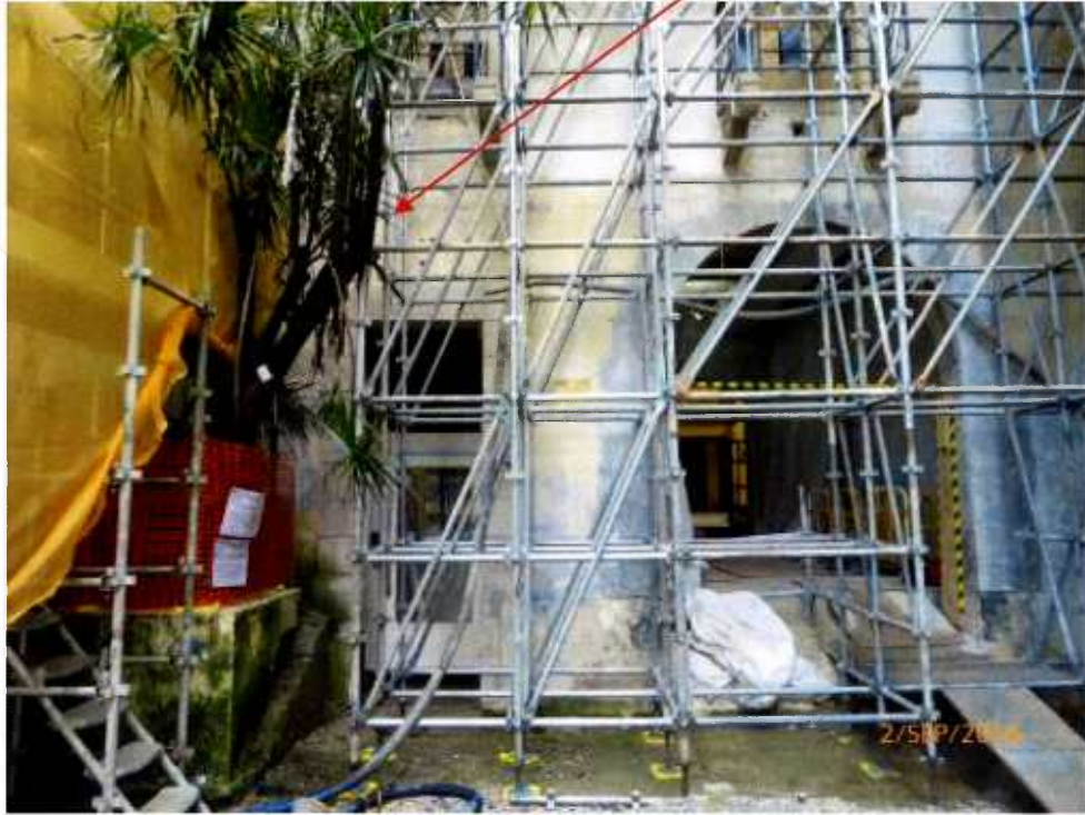
Fig. 10 Renovation works are in progress near Tree-11 .
