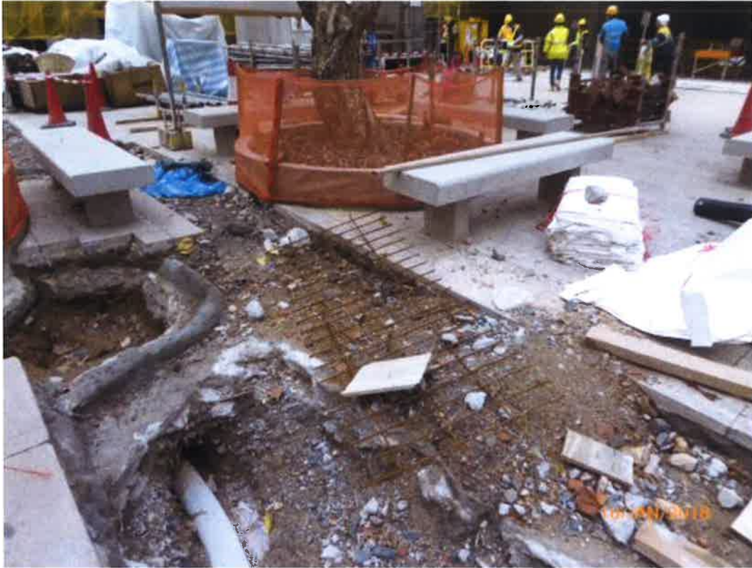
Fig. 10 The site near the planter seems to be re-constructed.
