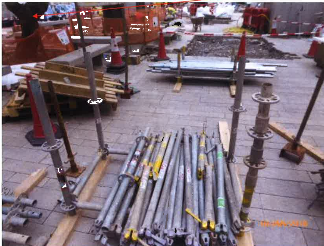
Fig. 11 Many construction equipment are placed near Tree-8.
