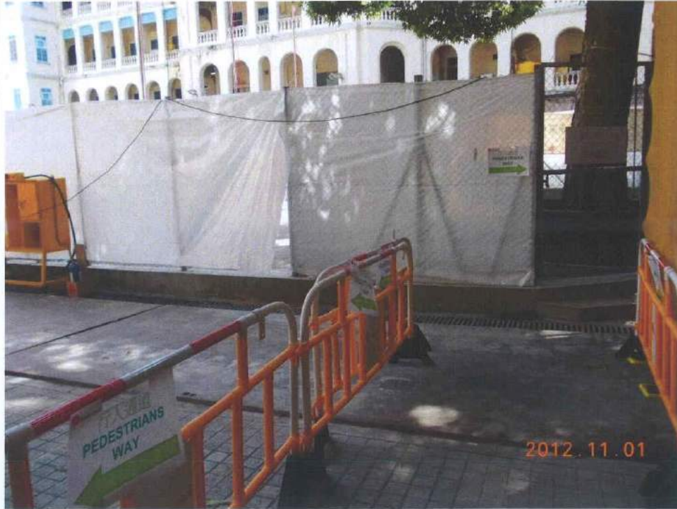
Fig. 6 The site outside the cordon zone is clean and tidy.
