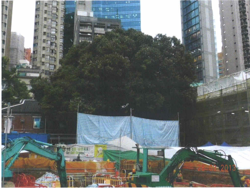
Fig. 8 Overall view of Tree-5 during inspection on 28 th March 2013.
