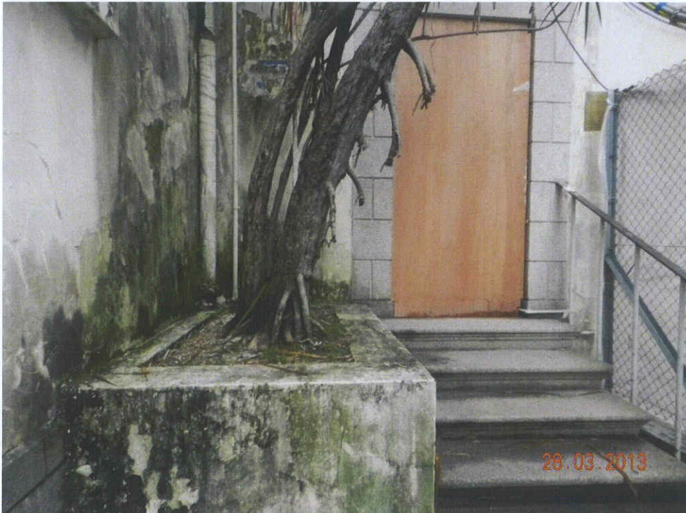
Fig. 3 The site is clean and tidy at the time of inspection.
