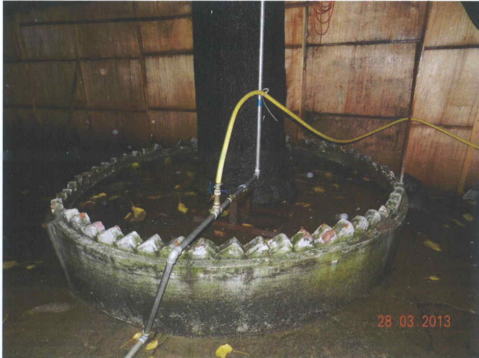
Fig 2. Cleanliness of the planter is acceptable.
