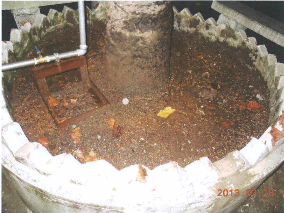
Fig 2. Cleanliness of the planter is acceptable.
