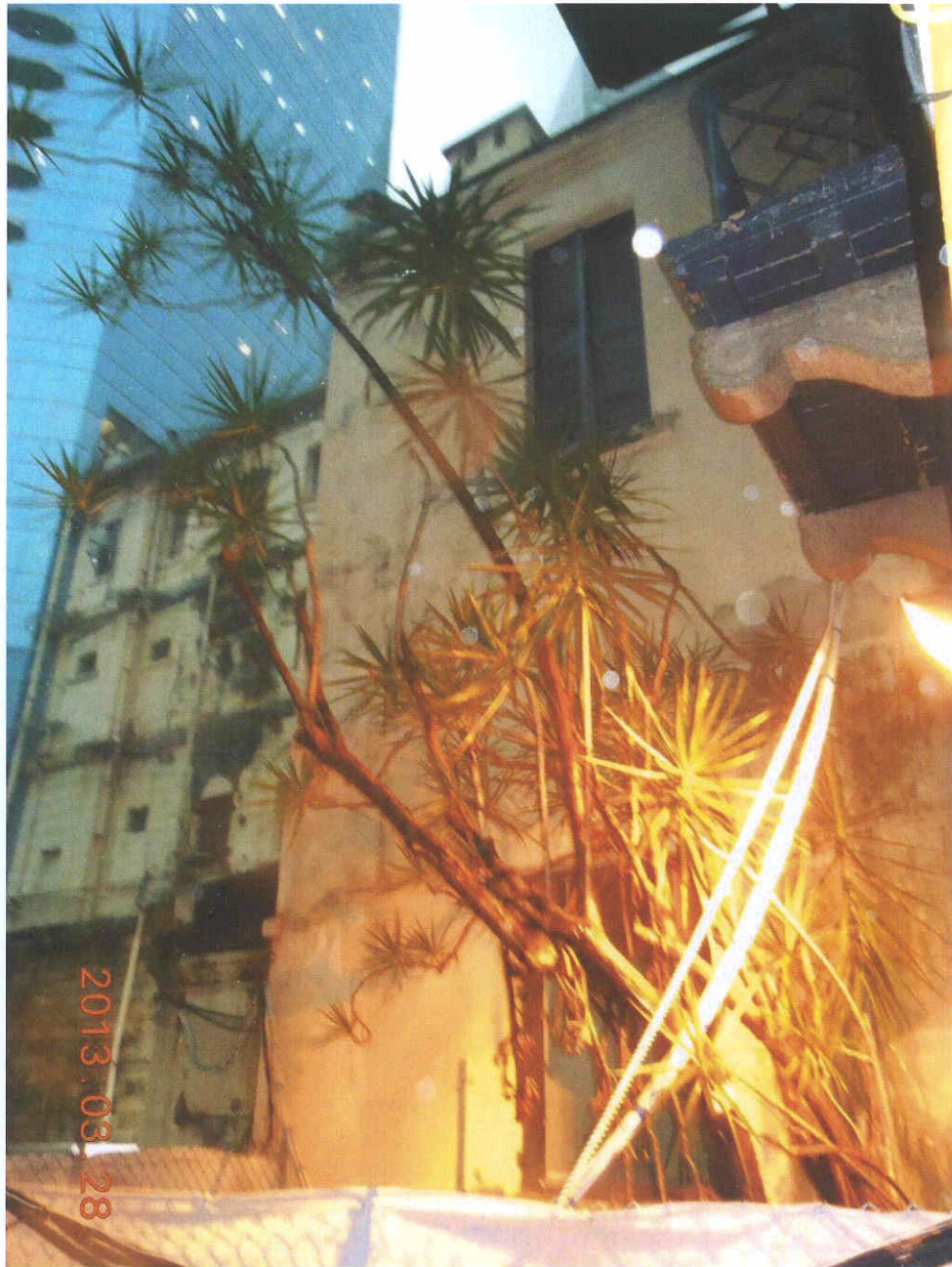
Fig. 6 Overall view of Tree-11 during inspection on 28 th March 2013.
