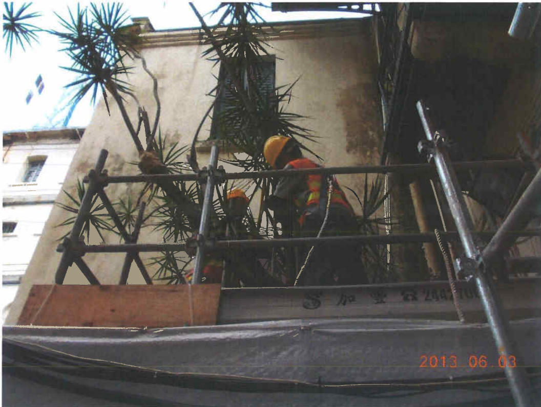
Fig. 3 Skilled workers use hessian cloth to wrap the tree.
