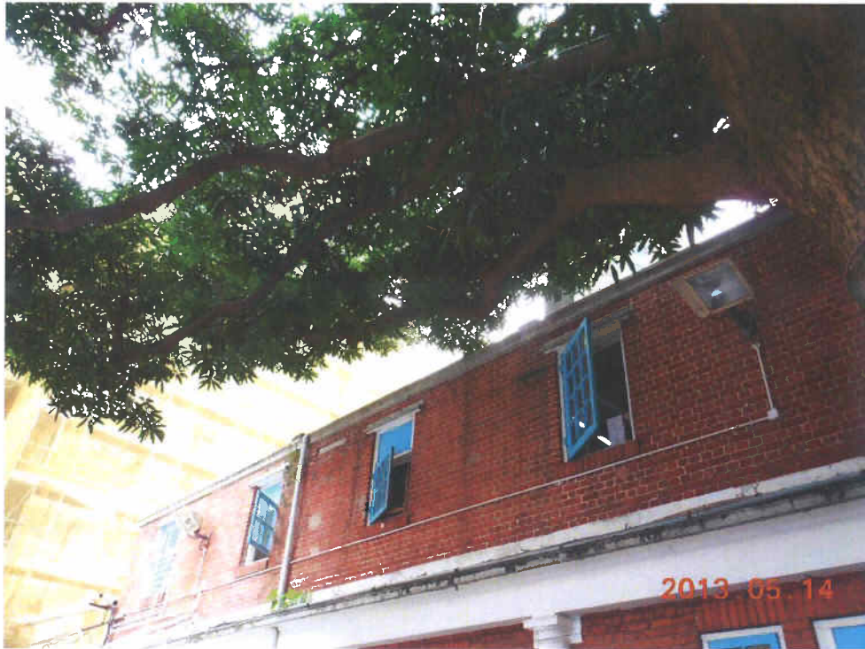
Fig. 4 Lower branches keep a reasonable distance from the building.
