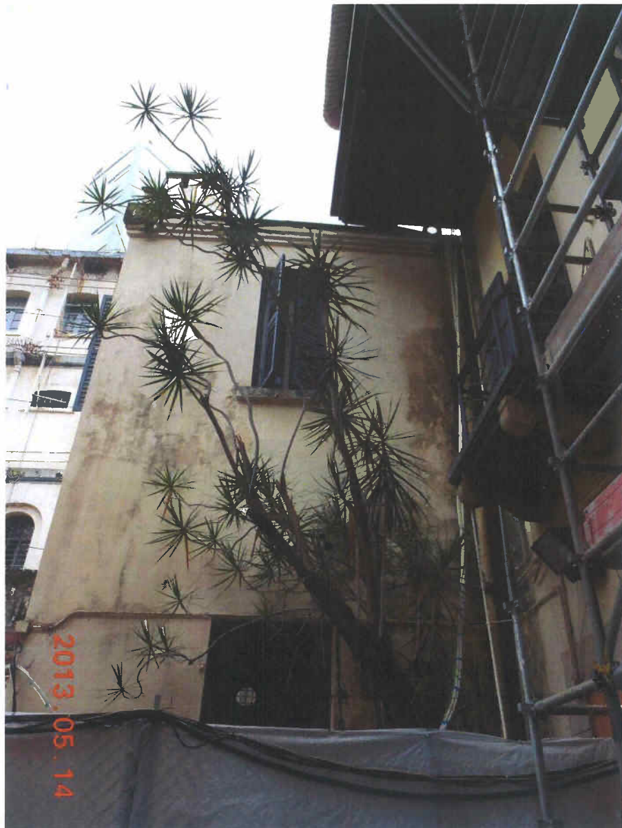
Fig. 8 Overall view of Tree-11 during inspection on 14 th May 2013.
