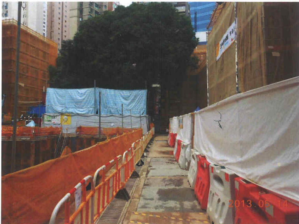
Fig. 7 The site outside the cordon zone keeps clean and tidy.
