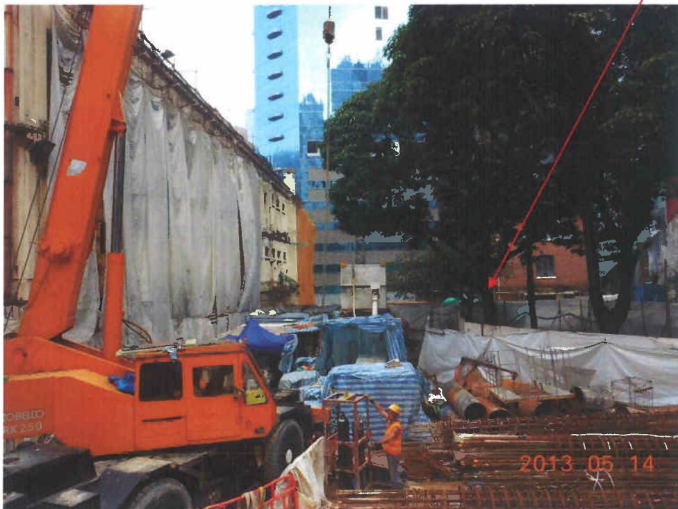
Fig. 5 Construction works are in progress outside the cordon zone. Tree-7
