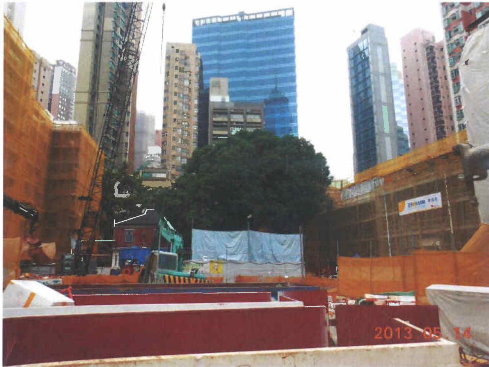
Fig. 8 Overall view of Tree-5 during inspection on 14 th May 2013.
