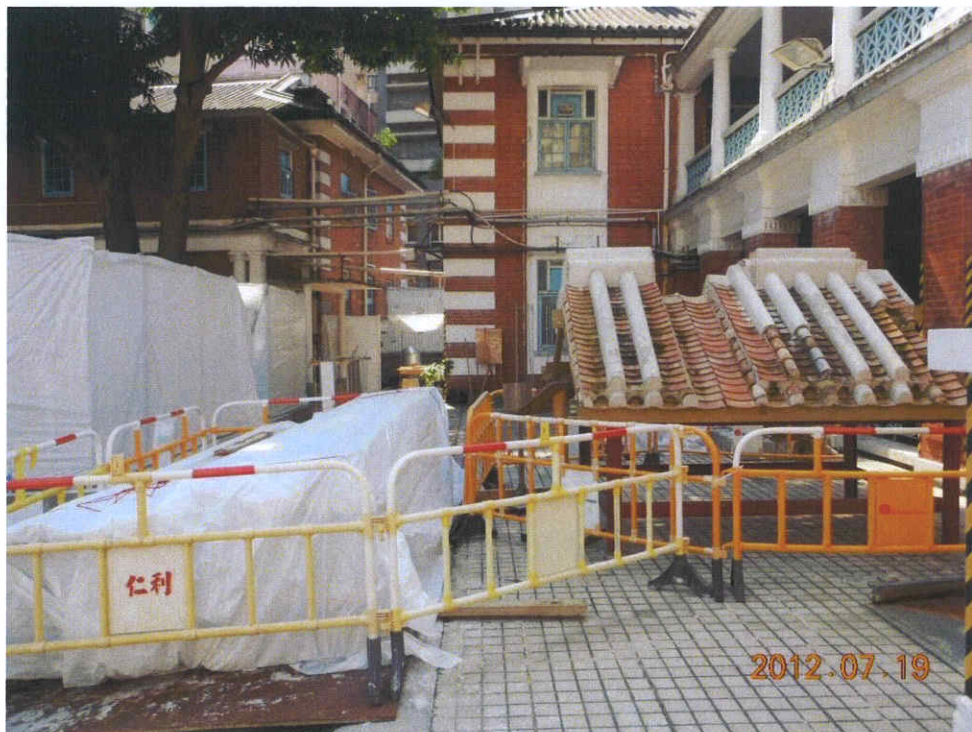
Fig. 7 Construction works o/s the cordon zone are in progress.
