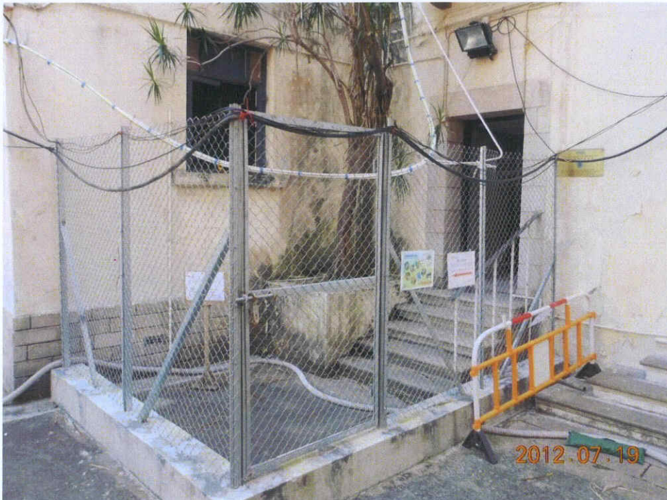
Fig. 5 The site inside the cordon zone is clean and tidy.
