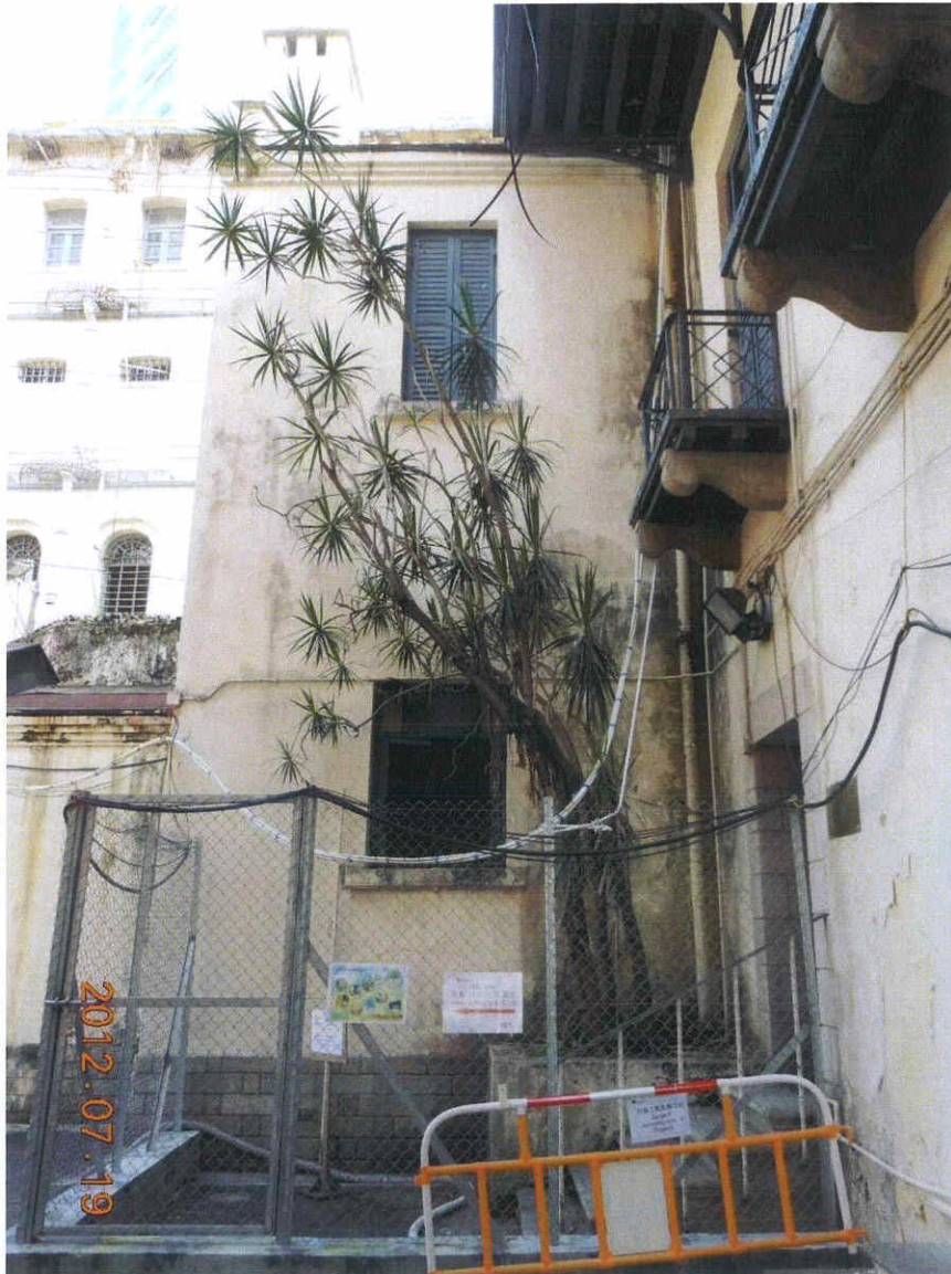
Fig. 6 Overall view of Tree-11 during inspection on 19 th July 2012.
