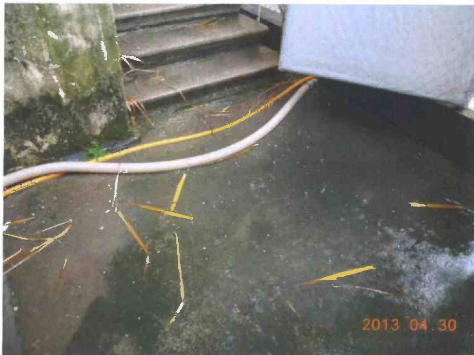
Fig. 3 Cleanliness of the site is acceptable.
