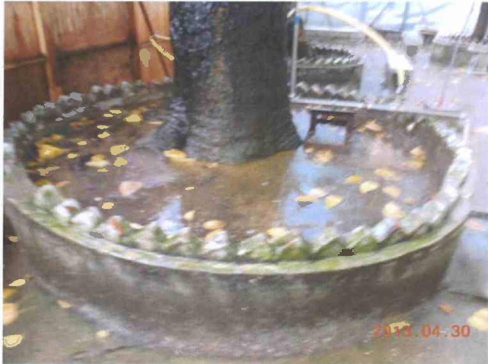
Fig 2. Cleanliness of the planter is acceptable.
