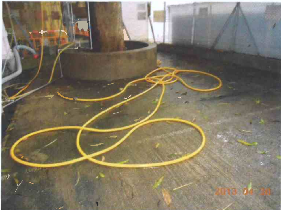
Fig. 3 Cleanliness of the site is acceptable.
