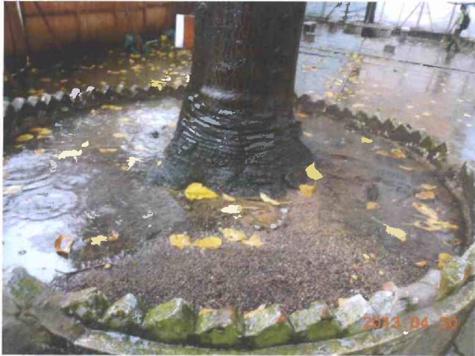
Fig 2. Cleanliness of the planter is acceptable.
