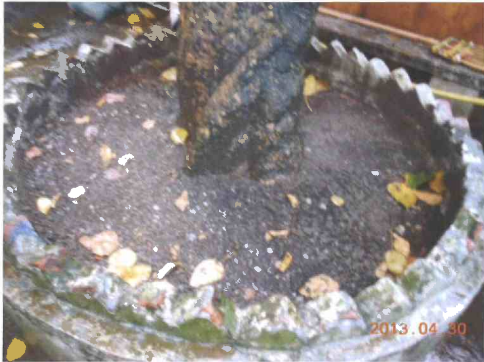
Fig 2. Cleanliness of the planter is acceptable.
