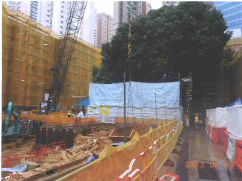
Fig. 6 Overall view of Tree-5 during inspection on 30 th April 2013.
