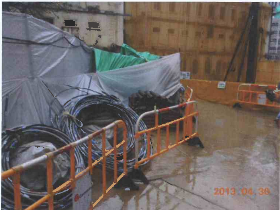
Fig. 5 It is raining at the time of inspection, the site outside the cordon zone is clean and tidy.
