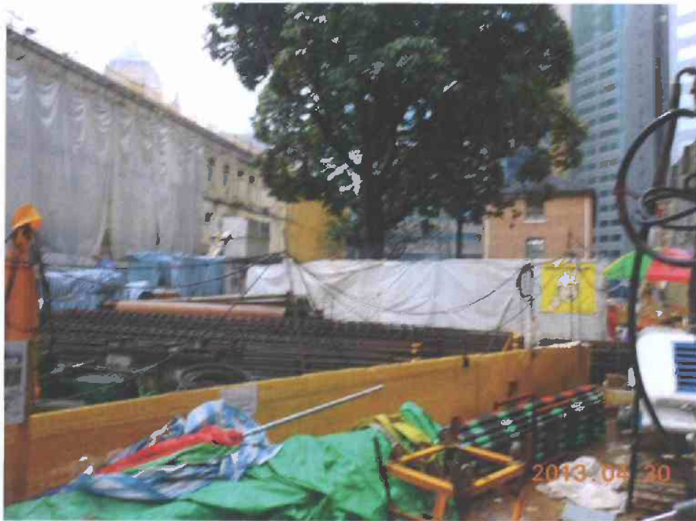
Fig. 4 Construction works are in progress outside the cordon zone.
