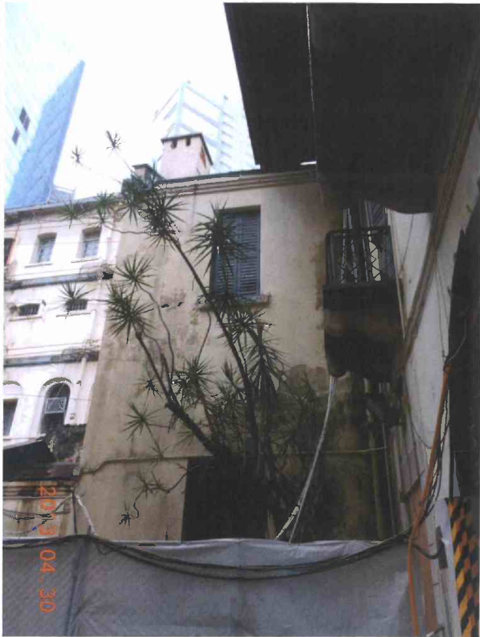
Fig. 6 Overall view of Tree-11 during inspection on 30 th April 2013.
