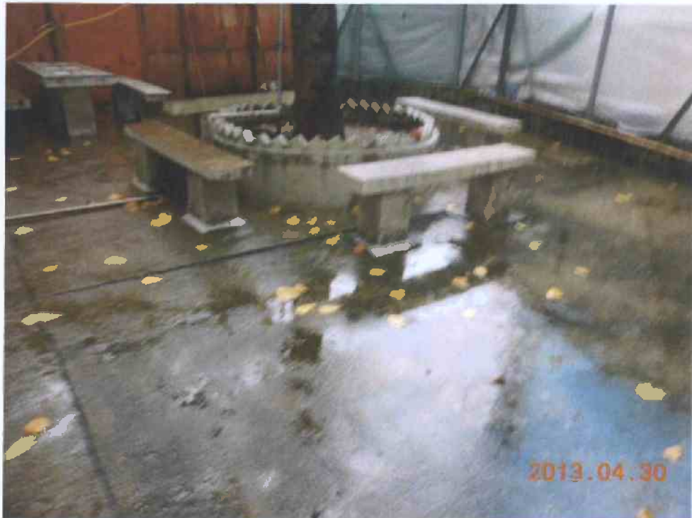
Fig 3 Cleanliness of the site is acceptable.
