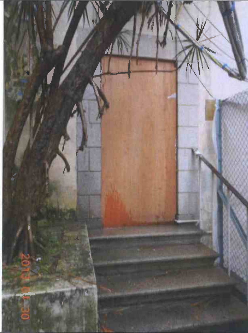
Fig. 4 A wooden partition has been installed at the nearby building.
