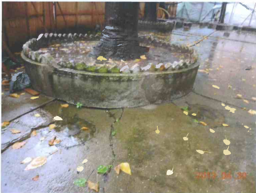
Fig. 3 Cleanliness of the site is acceptable at the time of inspection.
