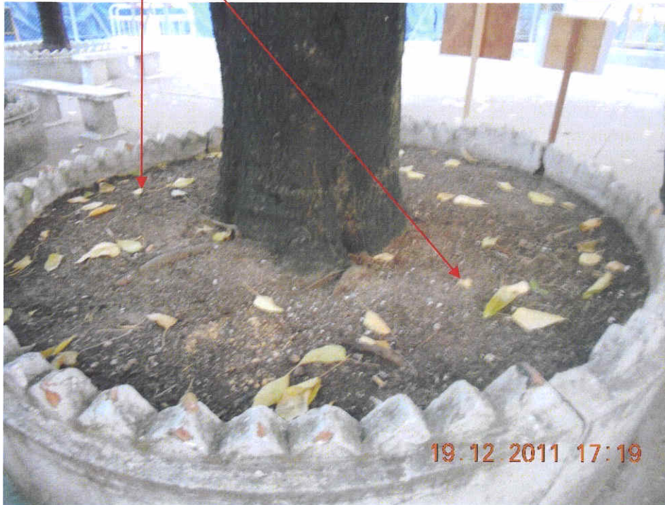
Fig 2. A few rubbish was found at the last inspection on 19 th December 2011.
