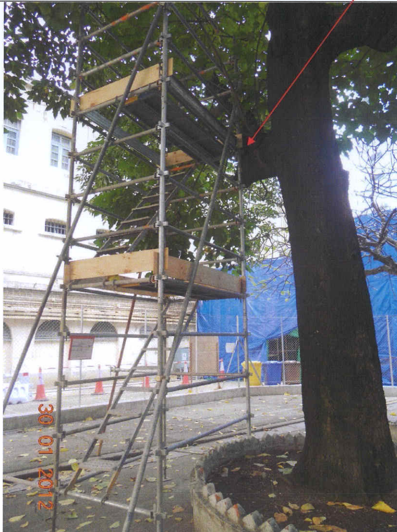
Fig. 5 A scaffold is too close to the tree, it will damage the bark easily .
