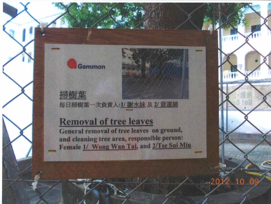
Fig. 5 Appropriate notice displays in front of the cordon zone.
