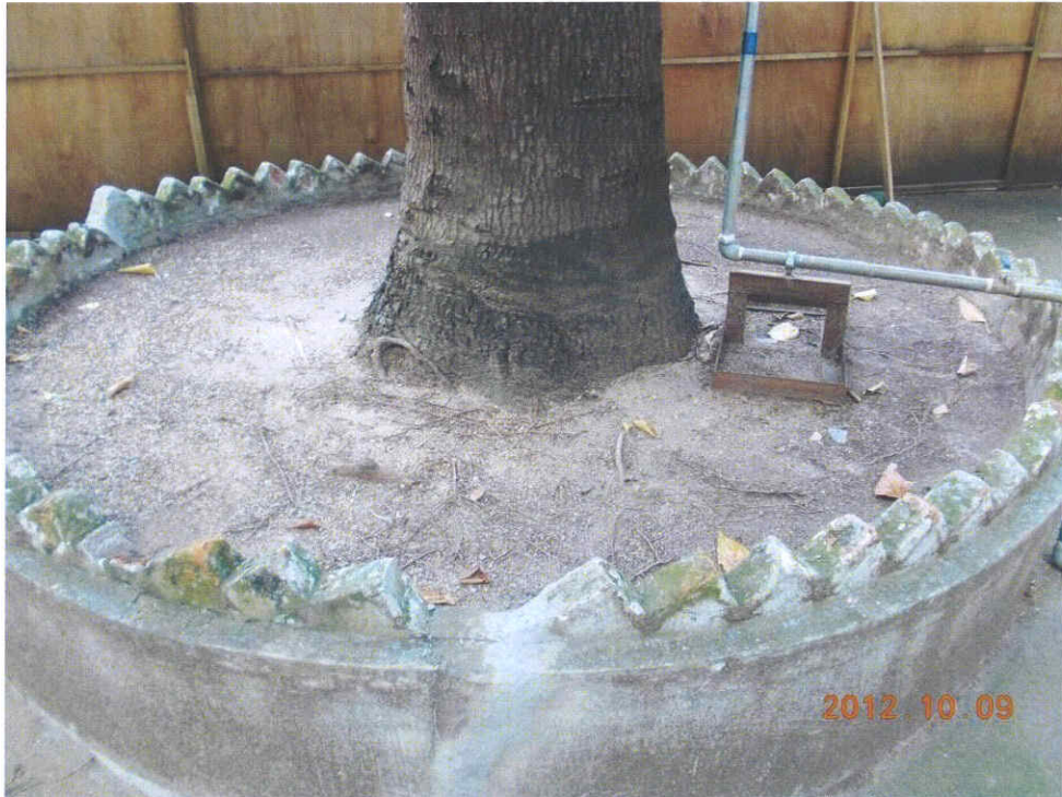
Fig 2. The planter is clean and tidy during inspection on 9 th Oct. 2012.
