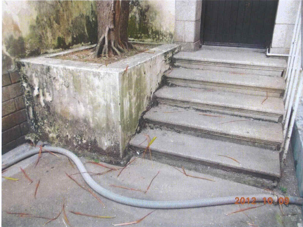
Fig. 4 Cleanliness of the site is acceptable.
