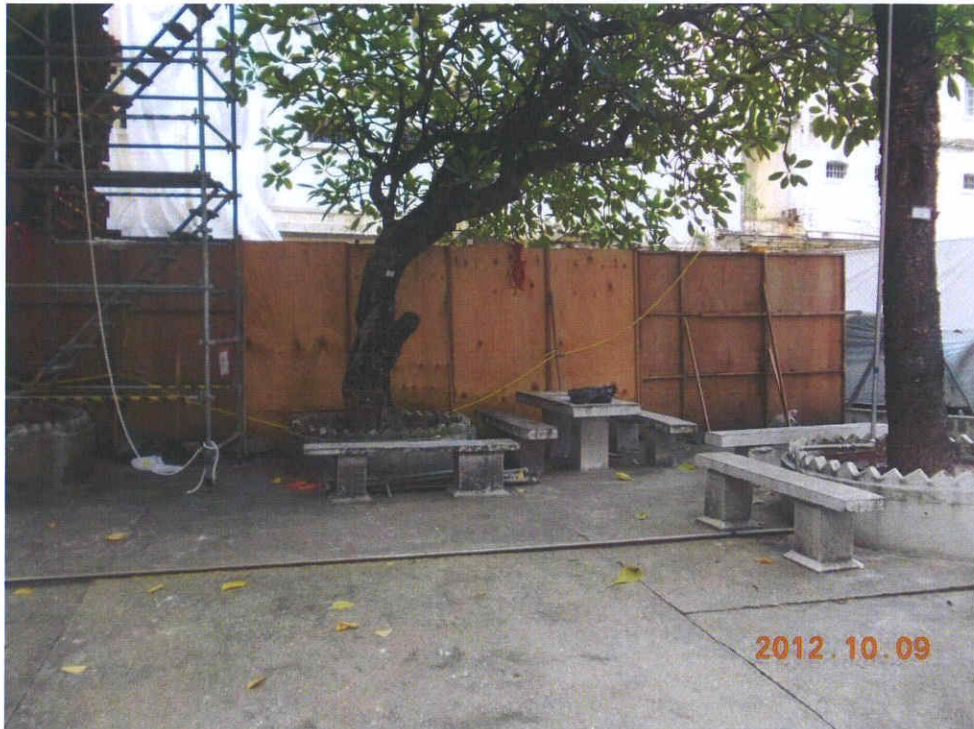
Fig. 3 Cleanliness of the site is acceptable.
