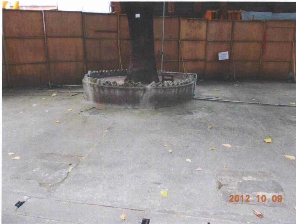
Fig. 4 The site inside the cordon zone is clean and tidy.
