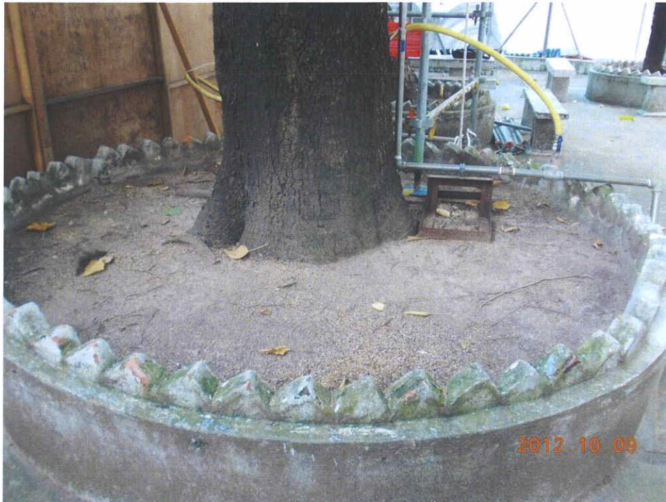
Fig 2. The planter is clean and tidy at the time of inspection.
