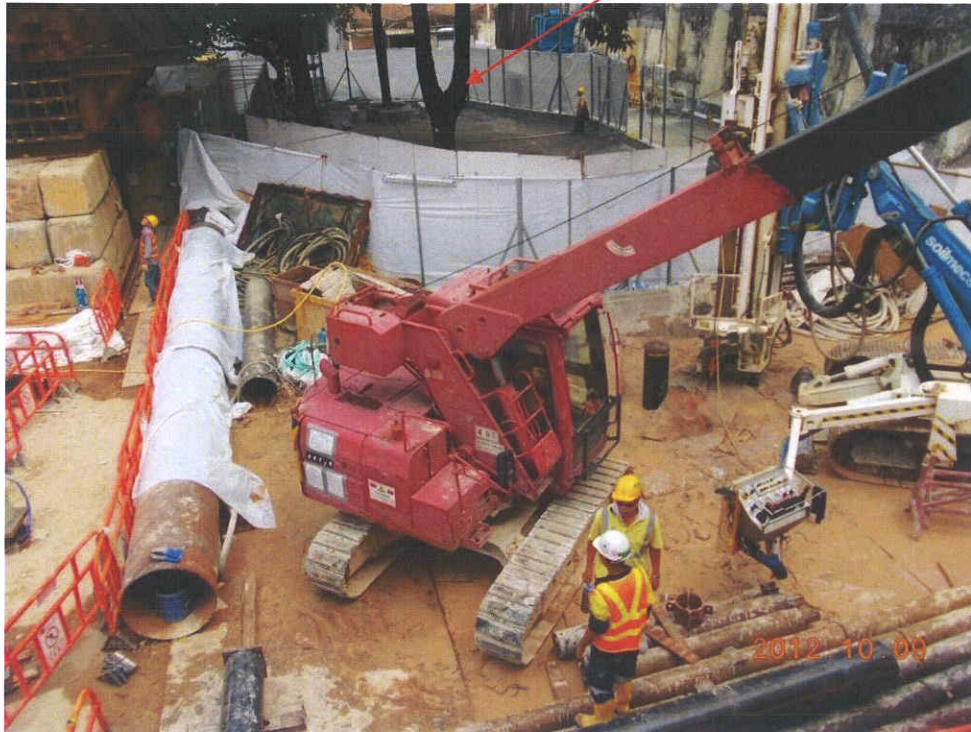
Fig. 8 Construction works are in progress near Tree-6.
