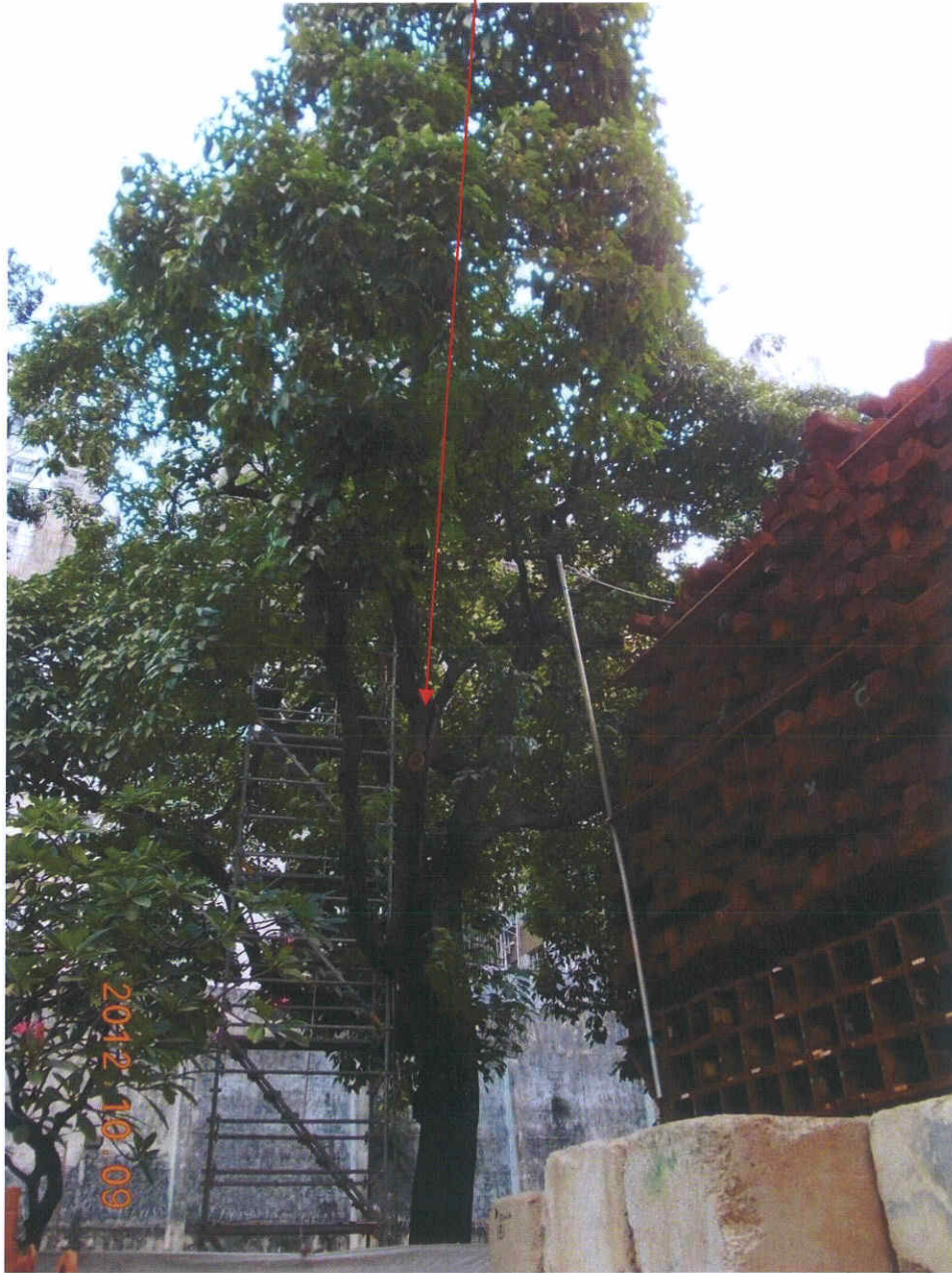
Overall view of Tree-7 during inspection on 9 th October 2012.
